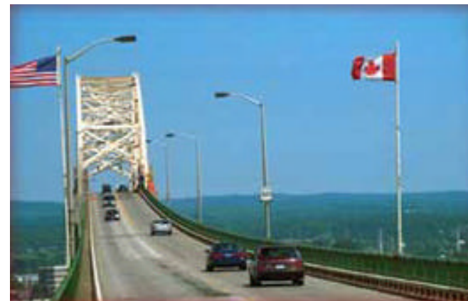
Source: Michigan Department of Transportation
