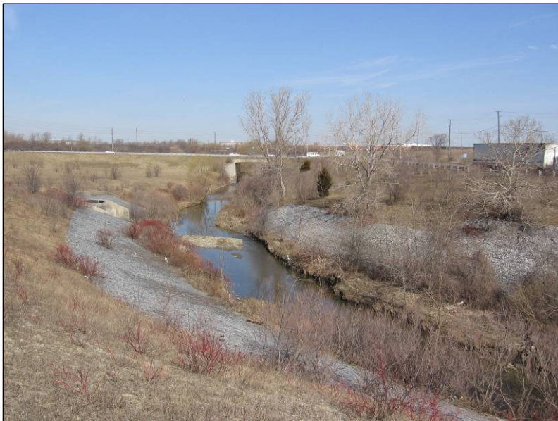
Mimico Creek proposed spur line crossing location, facing northwest (upstream) towards the Zahavy Way bridge.
