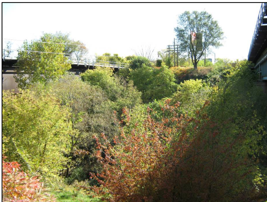
Black Creek crossing between rail bridges (Unit BC1) looking south showing early successional/regenerating vegetation.
