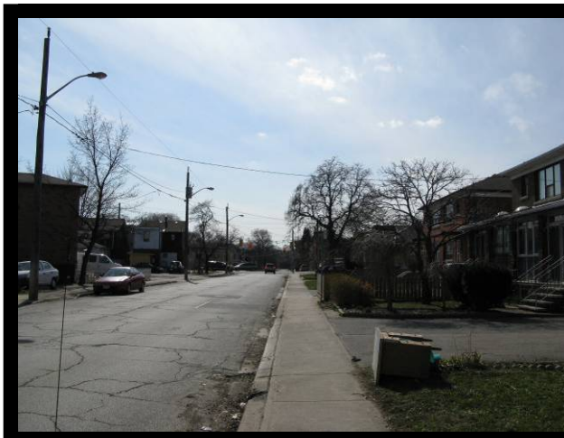
Residential land use west of the Dension Road at-grade crossing
