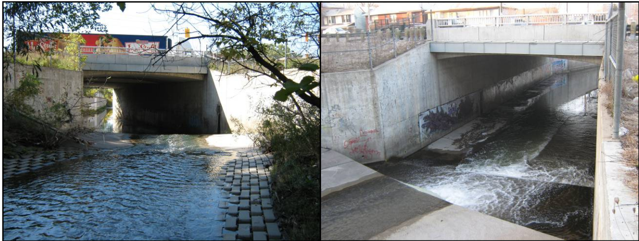
Black Creek – View west (downstream) from rail corridor crossing to Weston Road (note two-tiered grade control structure).
