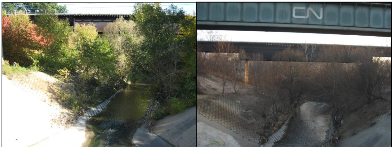
Black Creek – View east (upstream) from Weston Road towards the existing rail corridor crossing (in October 2008 and March 2009)
