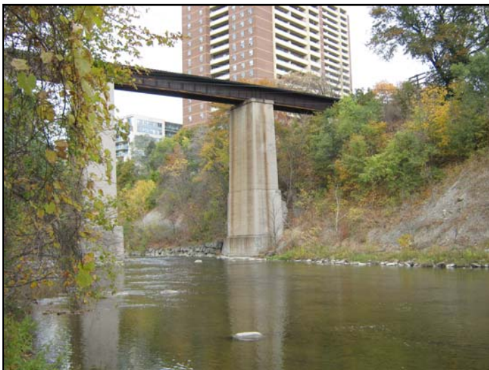
Humber River – View north to existing high level rail bridge.
