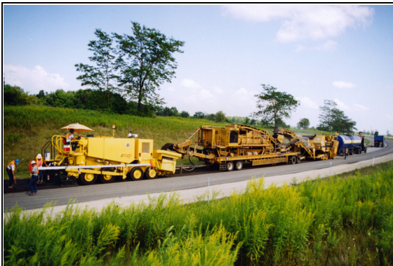
Photograph 3-4: Ontario CIR Project, 2000 This four piece recycling train consists of an emulsion tanker, milling machine, RAP crushing and screening unit and computerized pugmill/paver.
