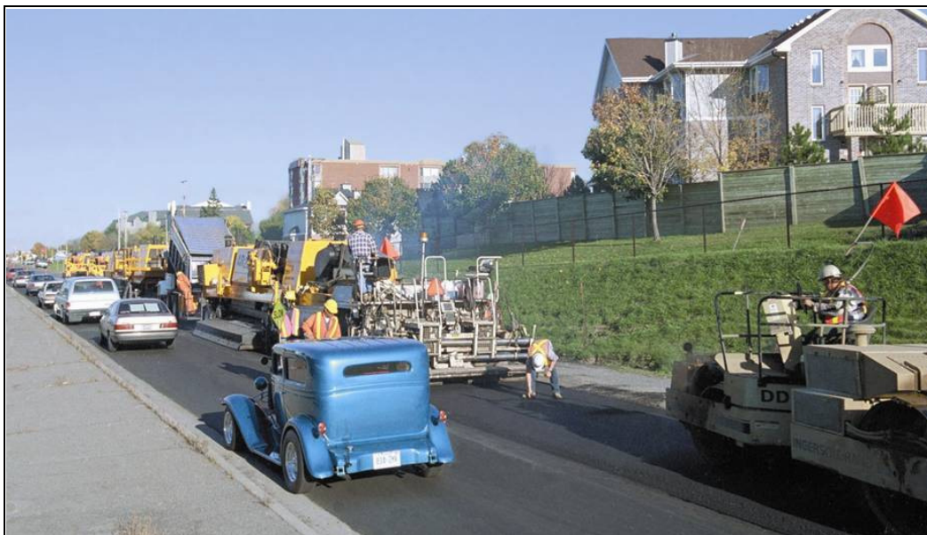
Photograph 3-3: Current HIR Remixing train rehabilitating a municipal roadway in a single pass, 2002
