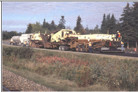
Photograph 3-5: Ontario CIR Project with cement slurry addition, 1999 Added to this CIR recycling train is a cement slurry tanker which gives the pugmill/paver the ability to add cement slurry to the mix.
