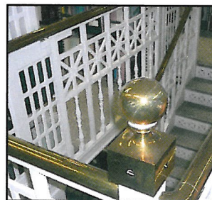
Brass finials top the newel posts on the original stack staircases. The risers are metal and the marble treads are of the same material as the stack decks.
