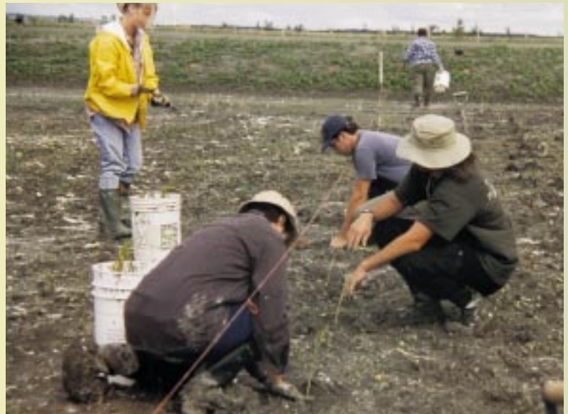
Fig. 2. Aquatic vegetation is critical to the success of a wetland in treating wastewater. At the Alfred site, cattails and bulrushes were planted by hand and by seeding. The success of the two methods will be compared once the plants are established.
