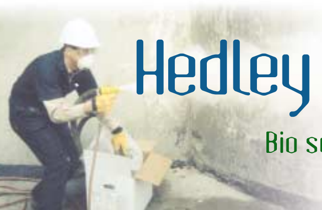
Fig. 1. Protect-It® structural application using compressed air gun. Effective pest management is critical in storage, shipping and processing facilities.
