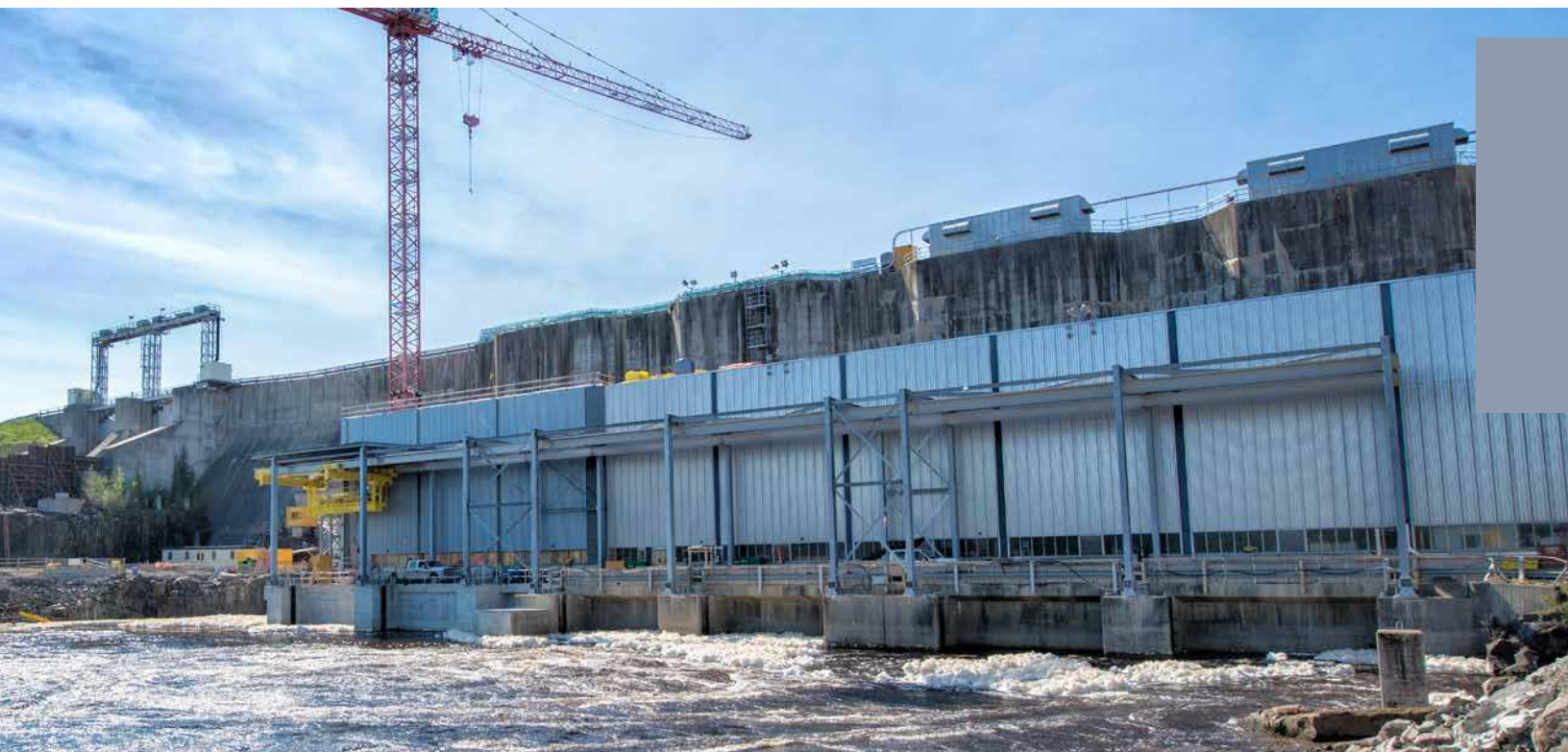
Construction de la centrale Kipling, Lower Mattagami
