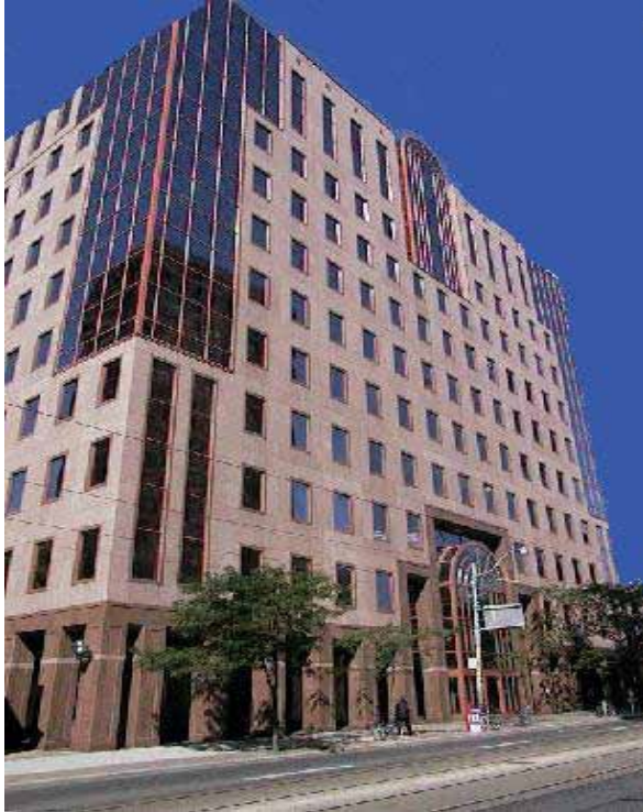
McMurtry-Scott Building, Toronto, Corporate Offices
