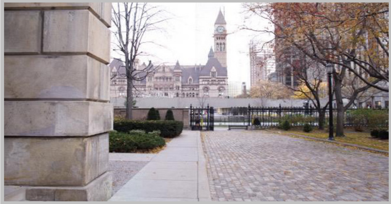
View of Toronto (Old City Hall) courthouse from the Court of Appeal for Ontario
