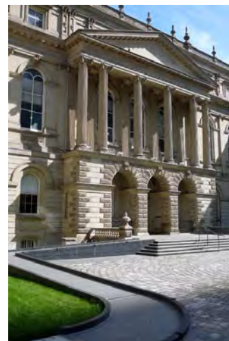
Osgoode Hall accessible ramp entrance
