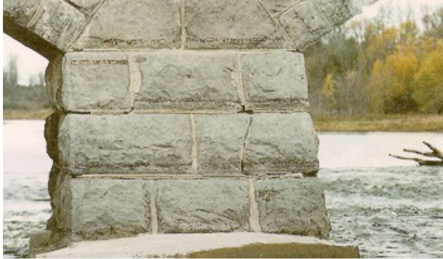
Figure 2.5.1 A Wide Crack Through the Stone in a Masonry Pier
