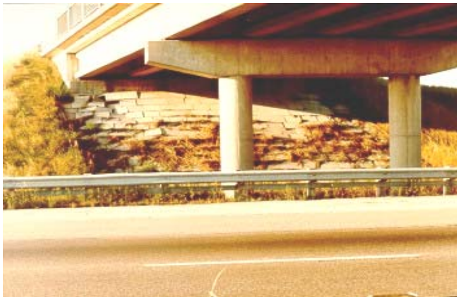
Figure 8.9(g) Precast Concrete Slope Protection
