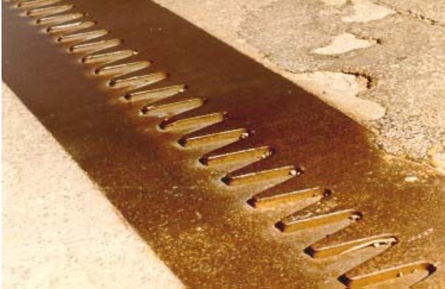
Figure 8.11(a) Finger Plate Expansion Joint
