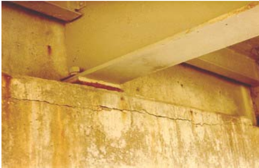
Figure 8.1(g) Concrete Ballast Walls
