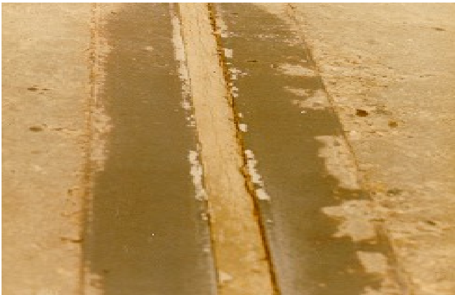
Figure 8.11(d) Ethylene Vinyl Acetate Seal
