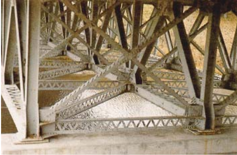
Figure 8.5(a) Sway Bracing and Bottom Lateral Bracing
