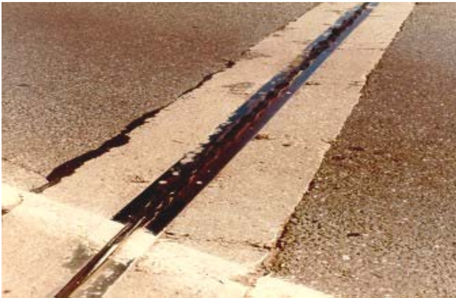
Figure 8.11(b) Compression Seal Joint
