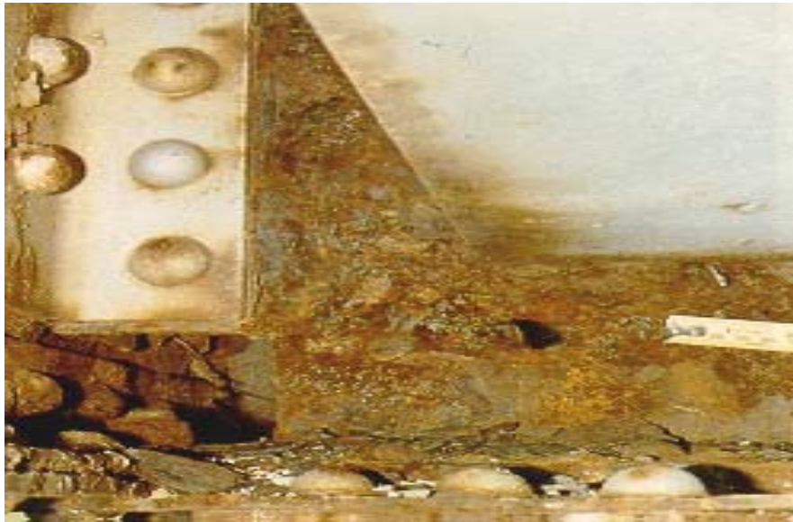
Figure 8.4(a) Floor Beam of Steel Through Truss
