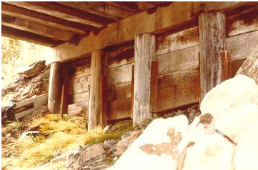
Figure 8.1(b) Wood Lagging - Abutment Wall
