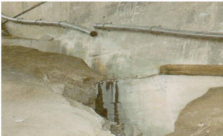
Figure 8.8(j) Drainage System
