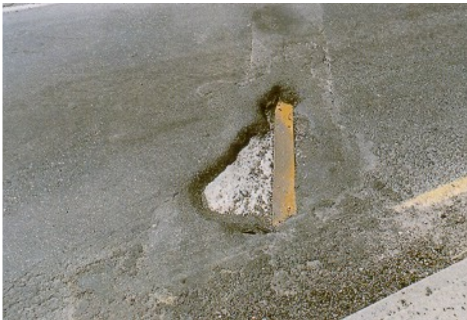
Figure 2.7.4 Severe Pothole
