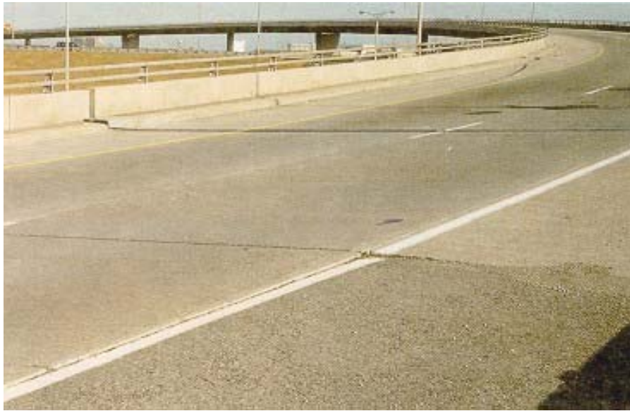
Figure 8.2(a) Concrete Approach Slab
