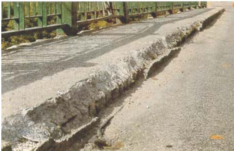
Figure 8.2(b) Concrete Sidewalk
