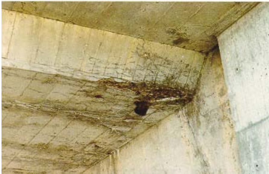
Figure 8.8(l) Thick Slab Soffit
