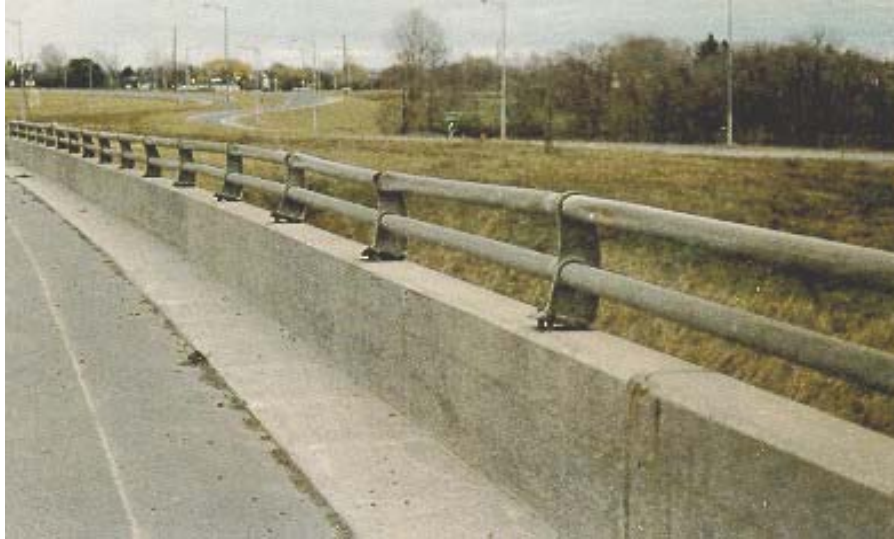
Figure 8.3(a) Parapet Wall
