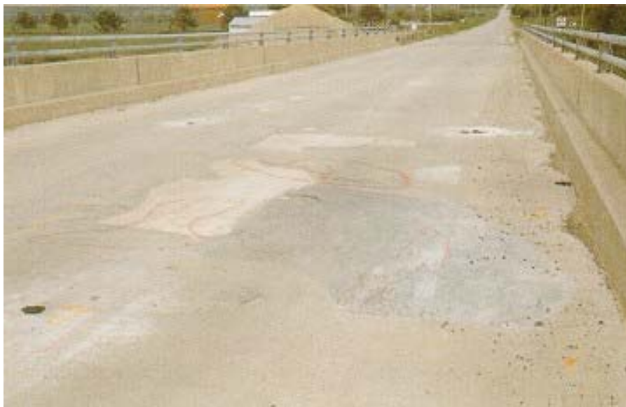
Figure 8.8(d) Concrete Deck
