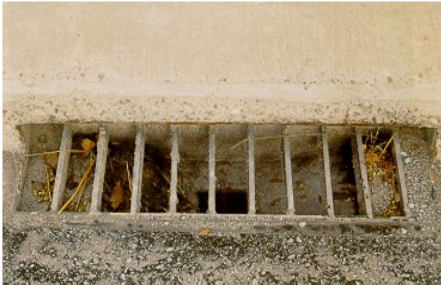
Figure 8.8(g) Deck Drain With Basin
