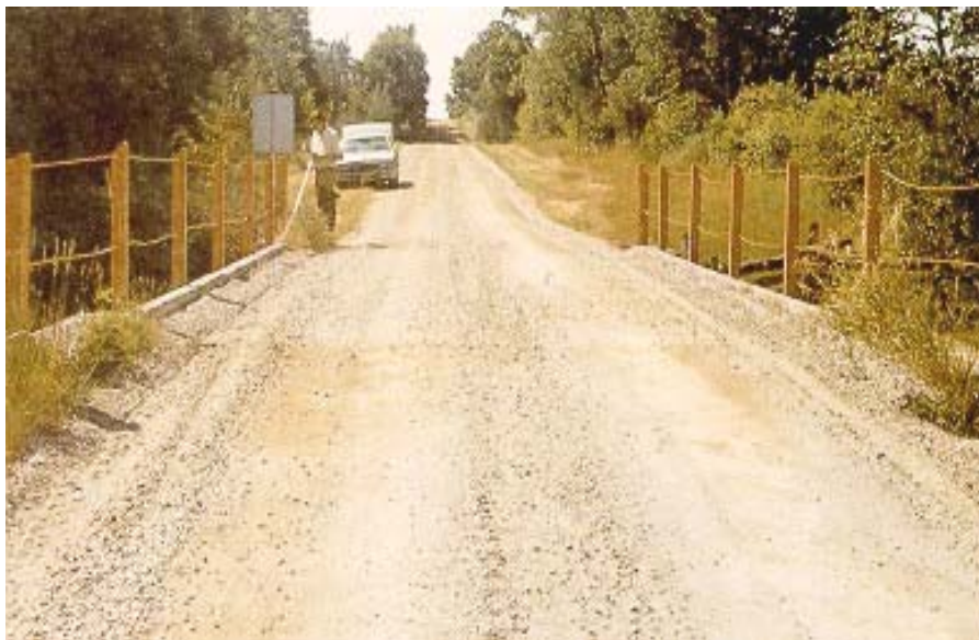
Figure 8.2(f) Gravel Approach
