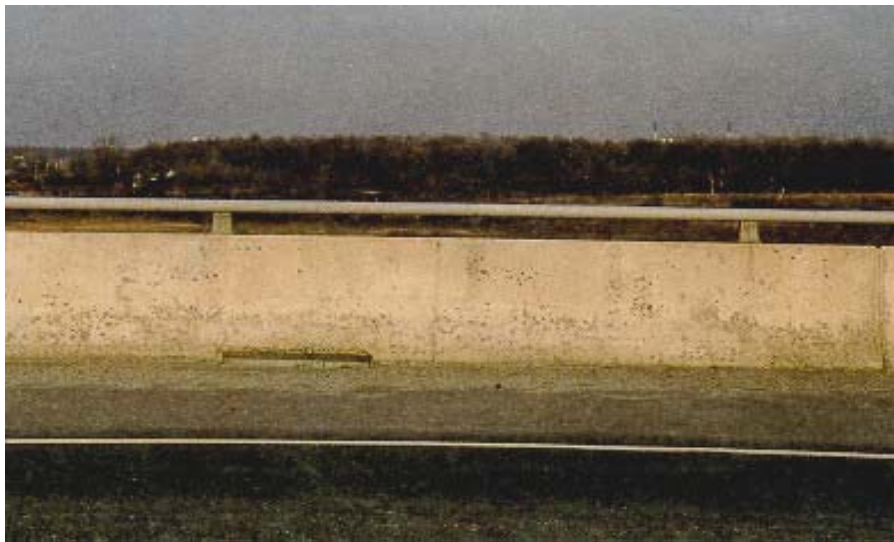
Figure 8.3(b) Barrier Wall
