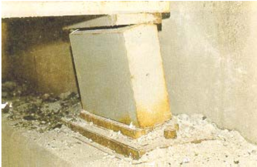
Figure 8.1(m) Steel Rocker Bearing
