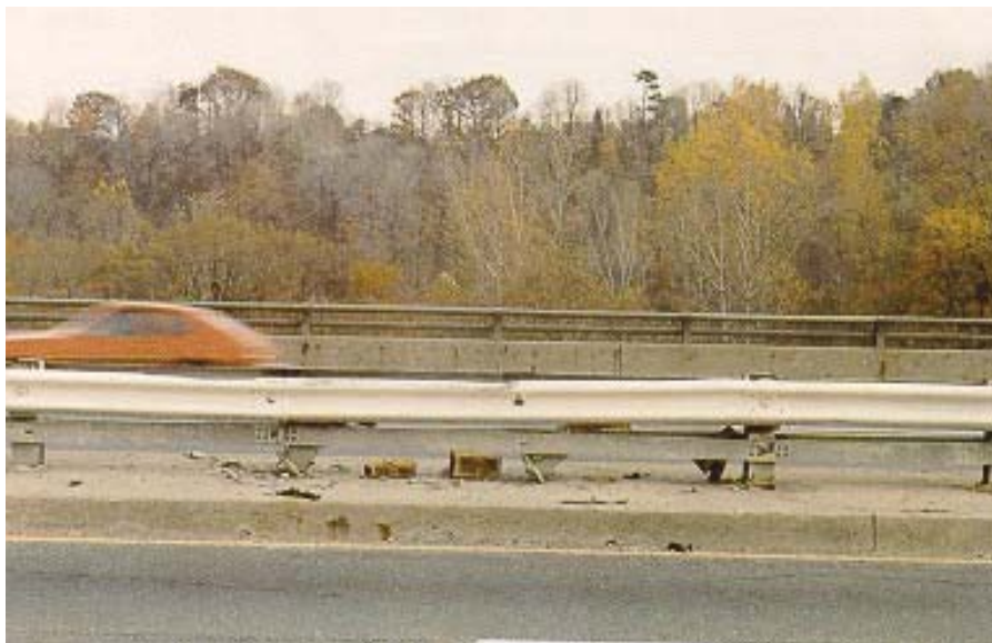
Figure 8.3(h) Steel Flex Beams
