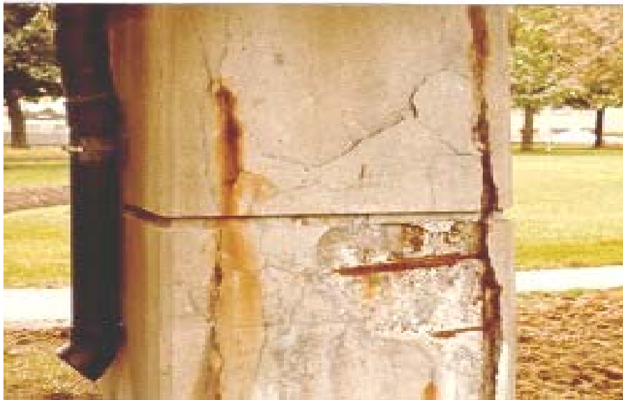
Figure 8.12(b) Concrete Pier Column
