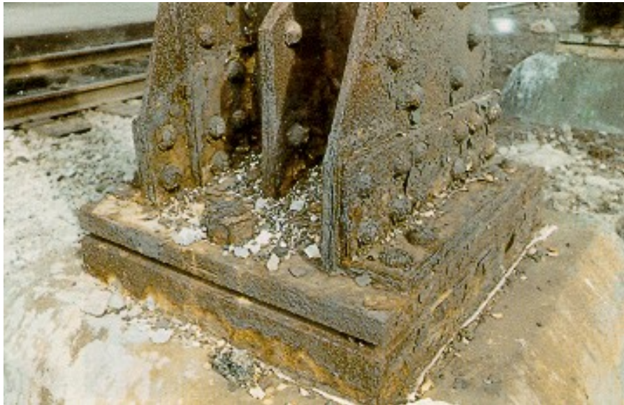
Figure 8.12(c) Steel Pier Bent Base
