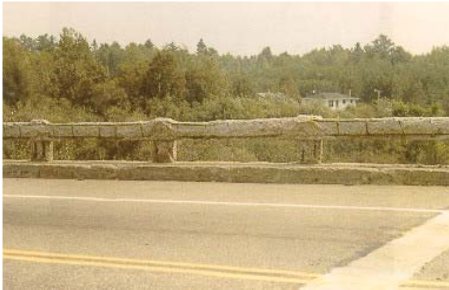
Figure 8.3(g) Concrete Guide Rail
