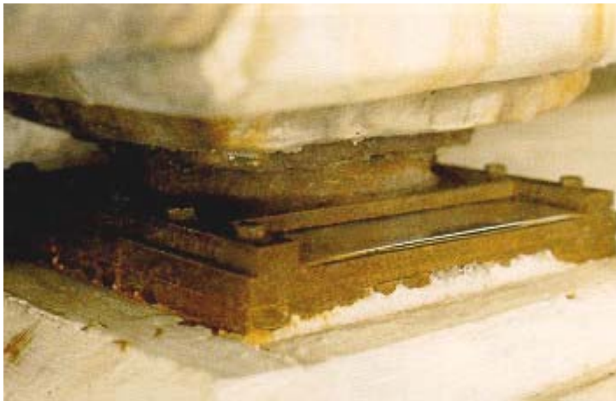
Figure 8.12(f) Disc Bearing
