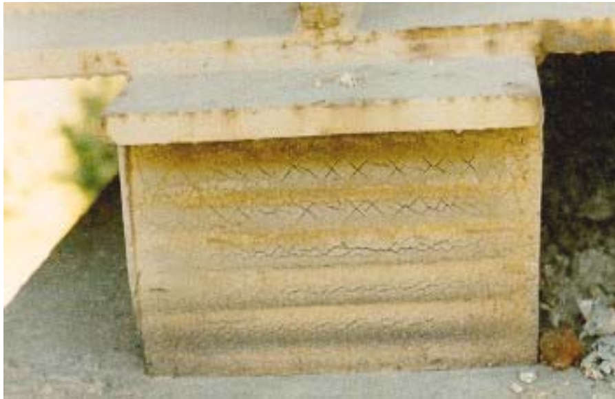
Figure 8.1(k) Laminated Elastomeric Bearing
