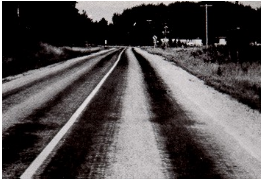
Figure 2.7.8 Slippery Surface
