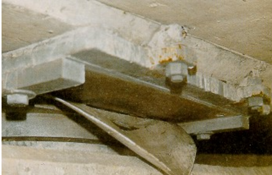
Figure 8.1(l) Pot Bearing
