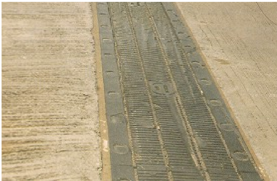
Figure 8.11(f) Rubber Cushion Joint
