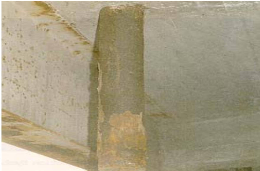
Figure 8.8(f) Steel Deck Drain
