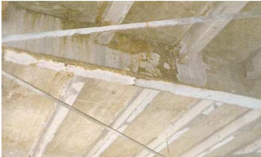
Figure 8.8(m) Soffit of a Thin Slab
