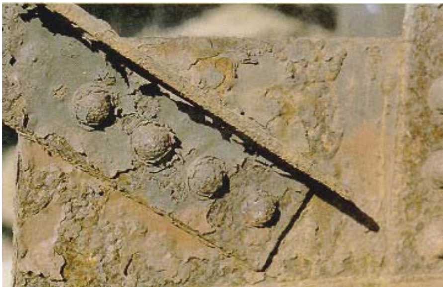
Figure 8.14(b) Sway Frame Connection.
