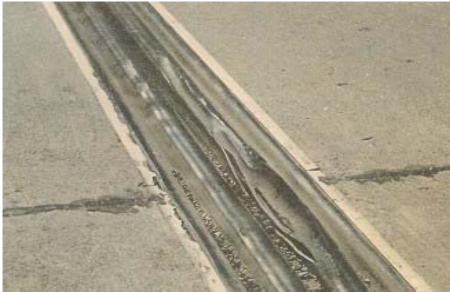
Figure 8.11(e) Multiple Seal Joint
