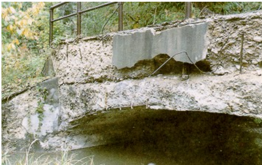
Figure 2.2.2 Very Severe Disintegration of Concrete in Exterior Face
