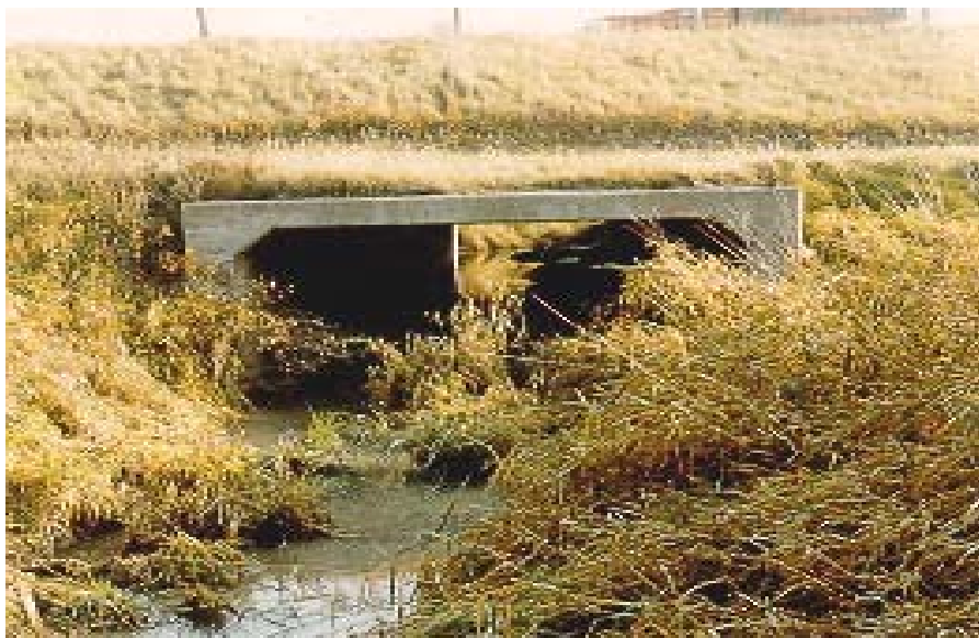
Figure 8.7(d) Concrete Open Footing Culvert
