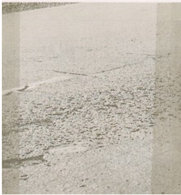
Figure 2.7.2 Severe Ravelling
