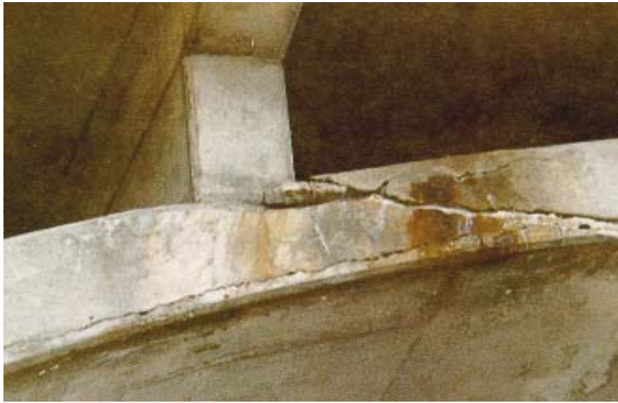
Figure 8.14(e) Concrete Spandrel Arch
