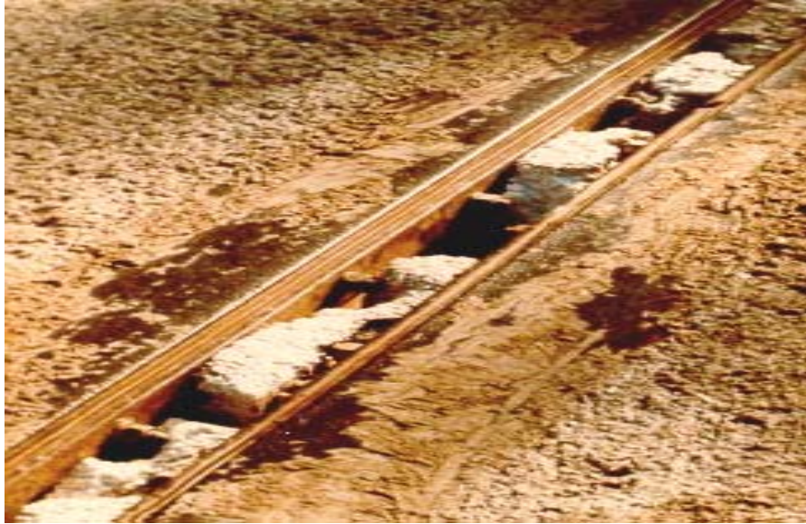
Figure 8.11(g) Horizontally Bolted Seal
