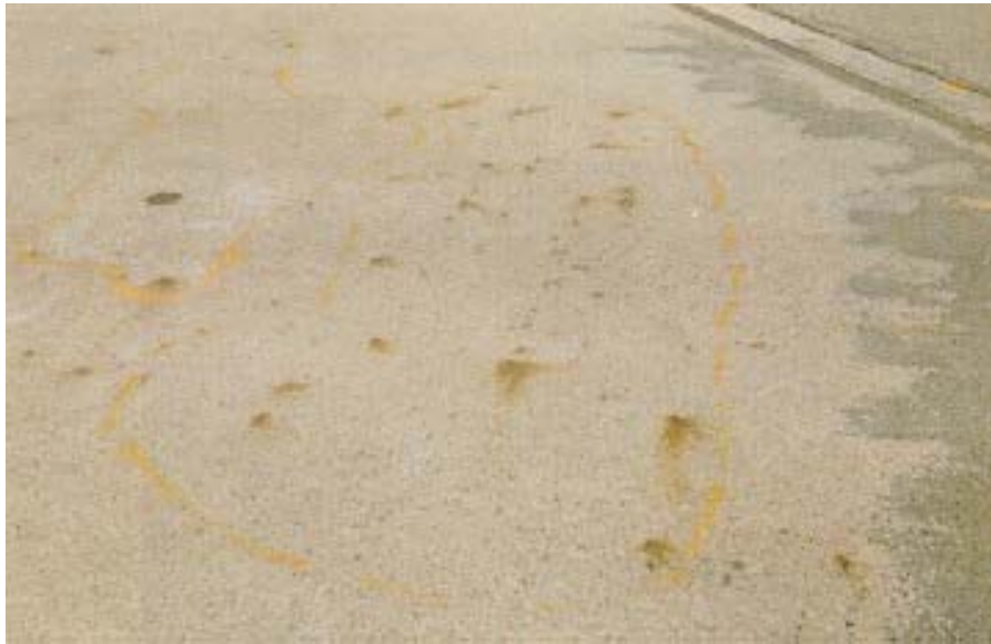
Figure 8.8(c) Concrete Deck
