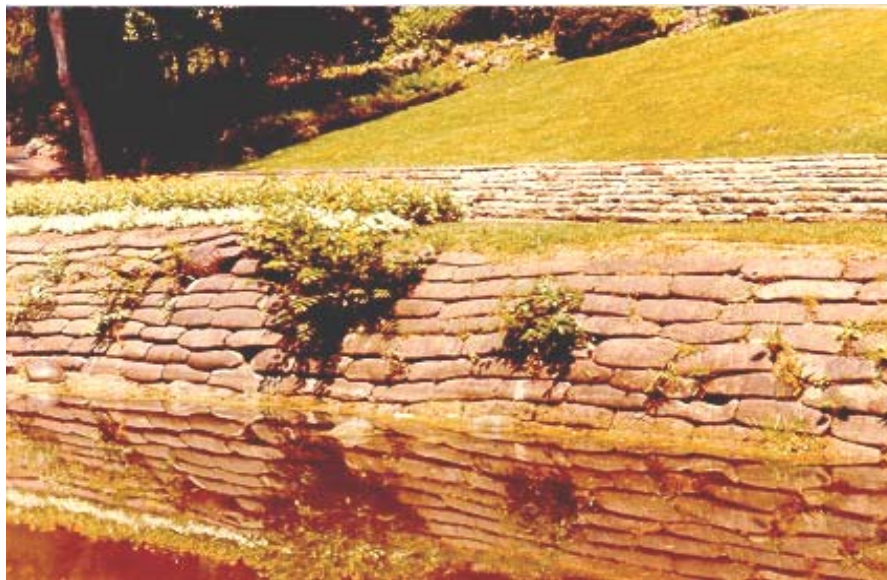
Figure 8.13(b) Bag Mortar Retaining Wall
