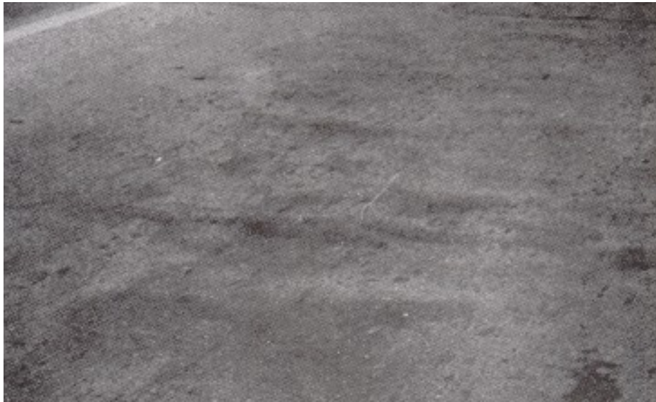
Figure 2.7.6 Severe Rippling
