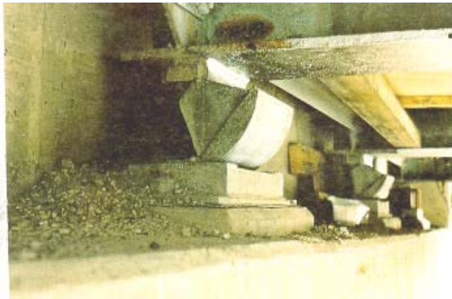
Figure 8.1(n) Steel Rocker Bearing
