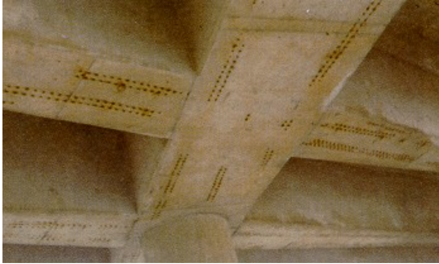
Figure 2.2.4(b) Light Stains on Concrete Surface Indicating Corrosion of Reinforcement
