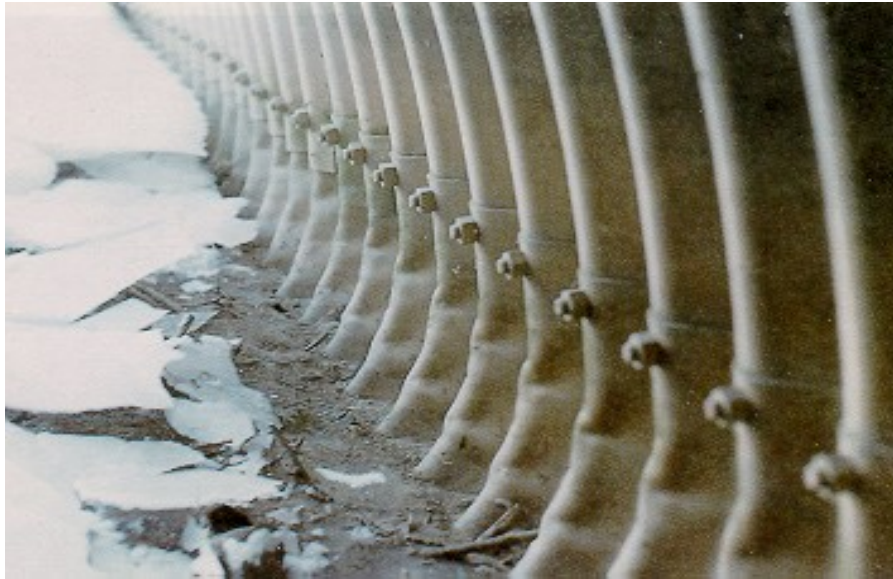
Figure 8.7(a) Multi-plate Pipe Arch
