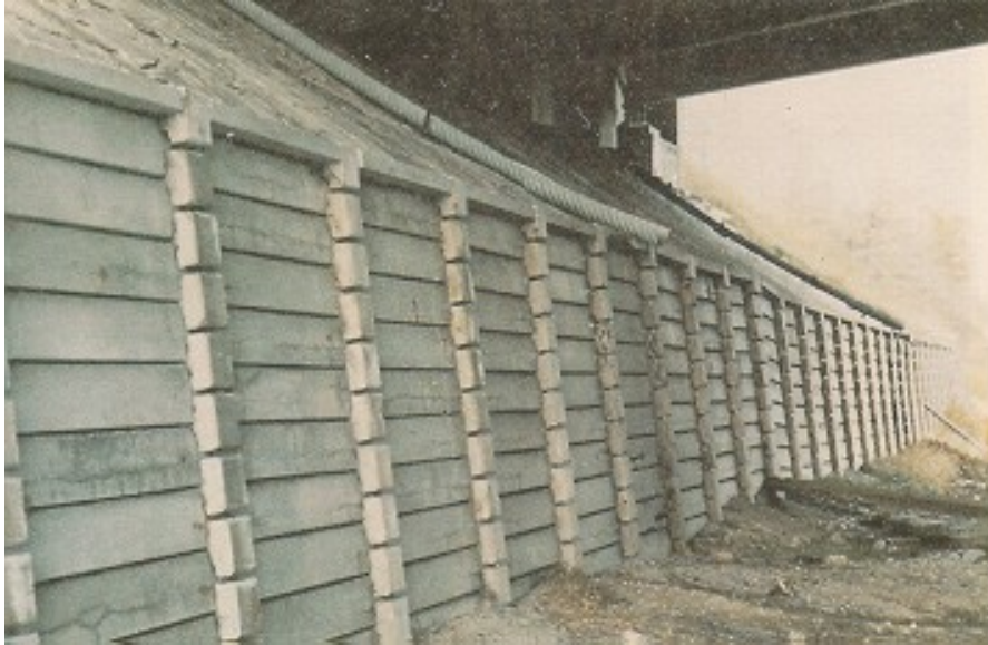
Figure 8.13(a) Precast Concrete Retaining Wall
