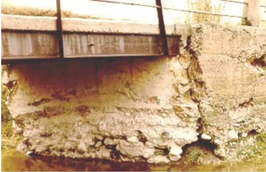
Figure 8.1(q) Concrete Wingwall
