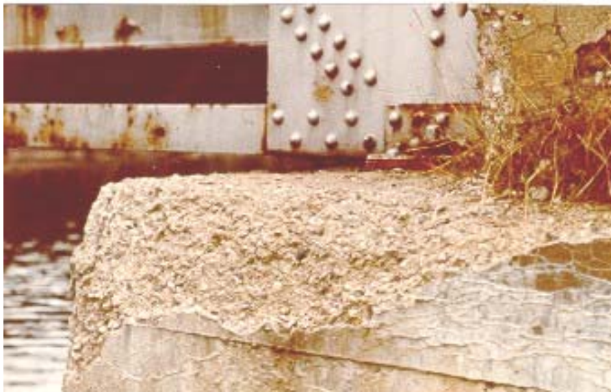
Figure 8.1(f) Concrete Abutment Wall
