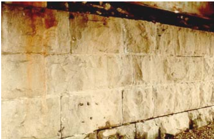
Figure 8.1(d) Masonry Abutment Wall
