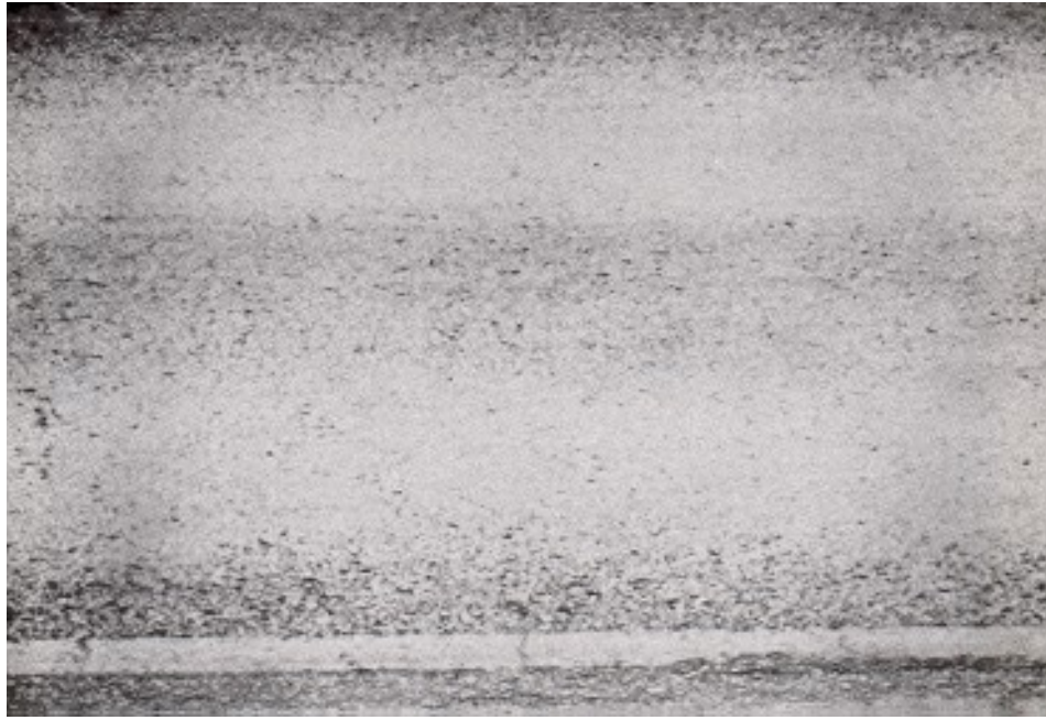
Figure 2.7.7 Severe Flushing
