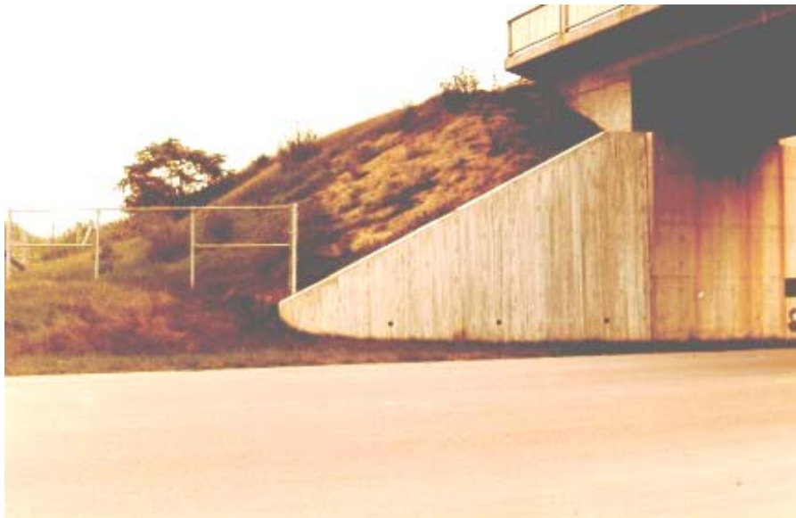
Figure 8.9(e) Grass Slope Protection
