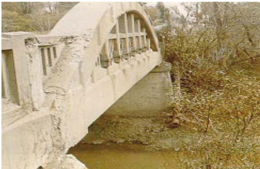
Figure 8.14(d) Concrete Bowstring Arch
