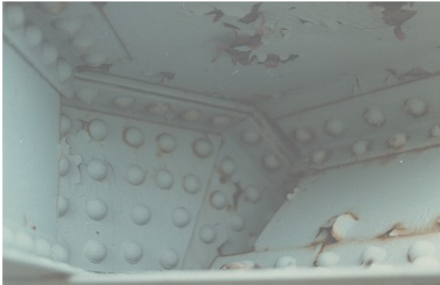
Figure 8.6(c) Connection of Primary Components
