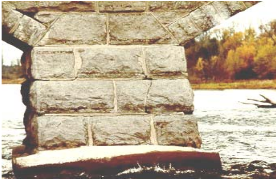
Figure 8.12(e) Masonry Pier
