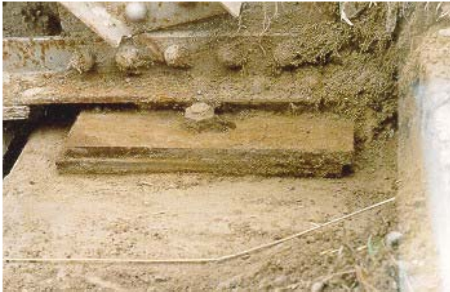
Figure 8.1(i) Steel Plate Sliding Bearing
