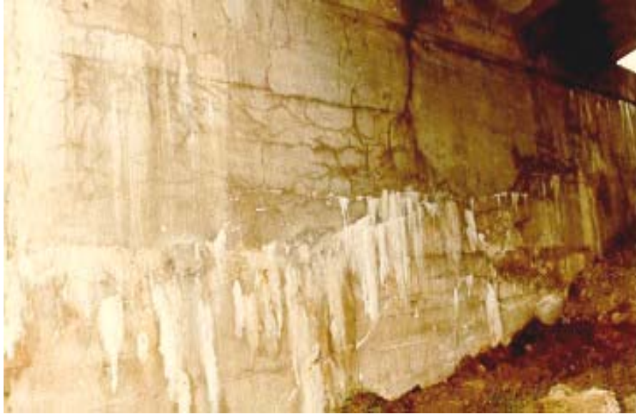
Figure 8.1(a) Concrete Abutment Wall
