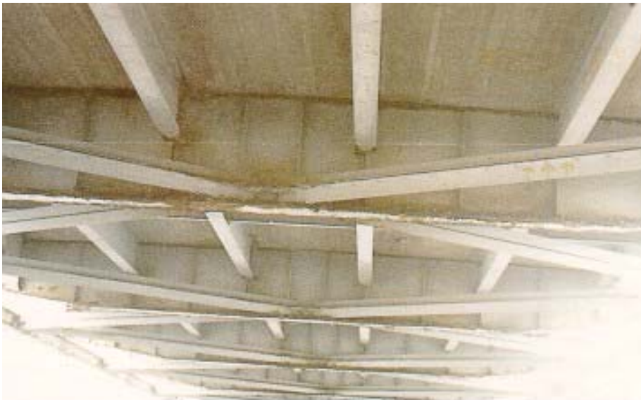
Figure 8.5(b) Bottom Lateral Bracing
