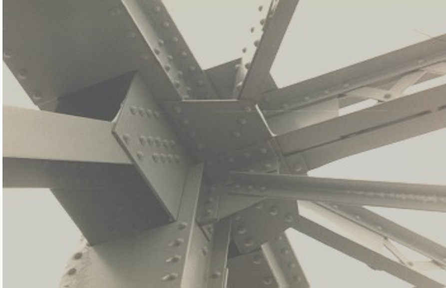
Figure 8.6(a) Through Truss - Connection of Primary Components
