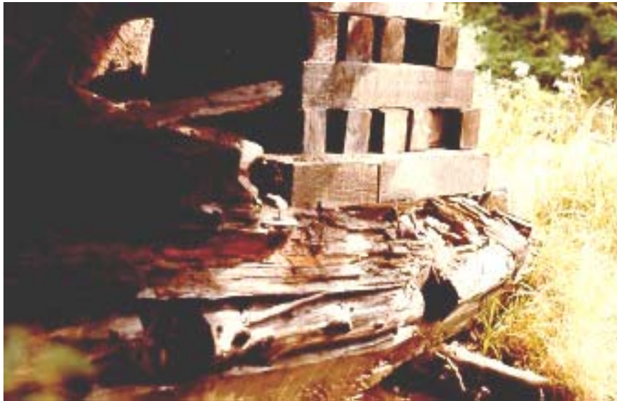
Figure 8.1(c) Wood Crib - Abutment Wall
