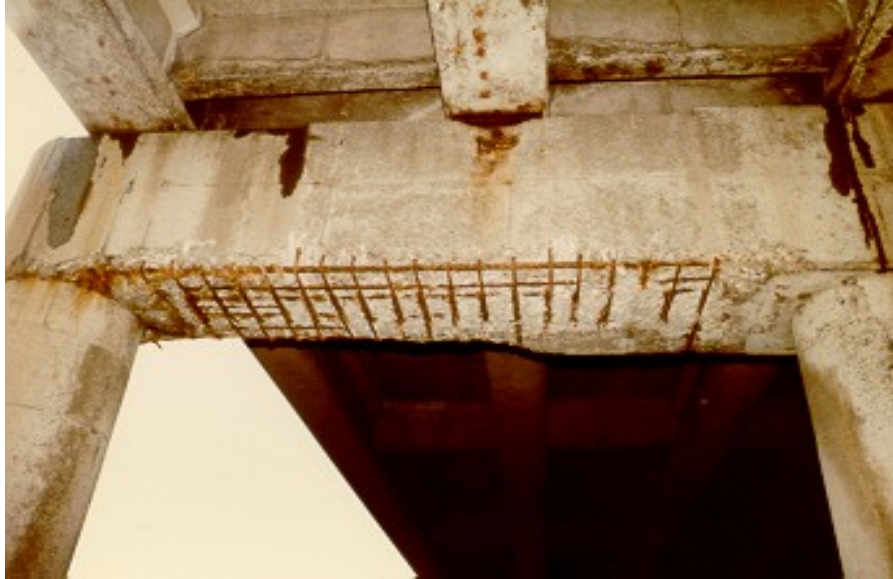
Figure 8.12(a) Concrete Pier Cap
