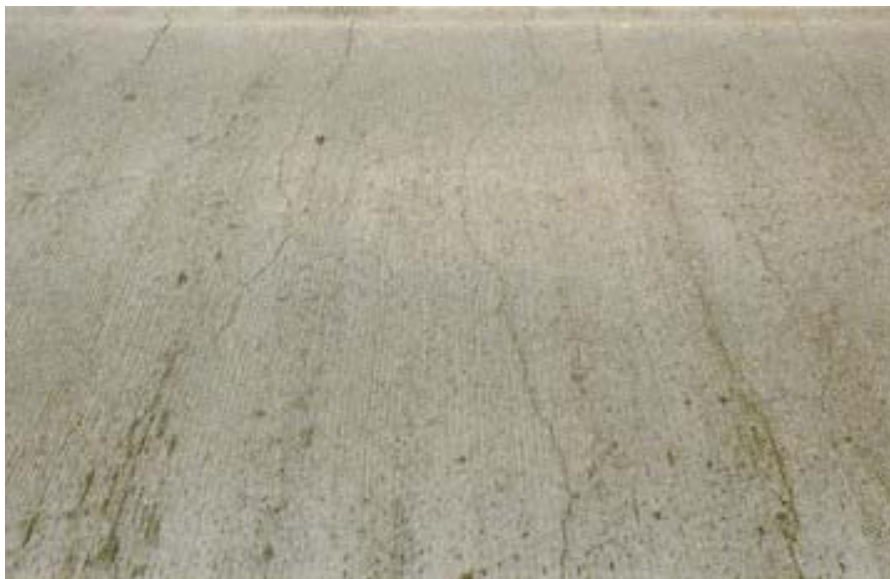
Figure 8.8(b) Exposed Concrete Deck
