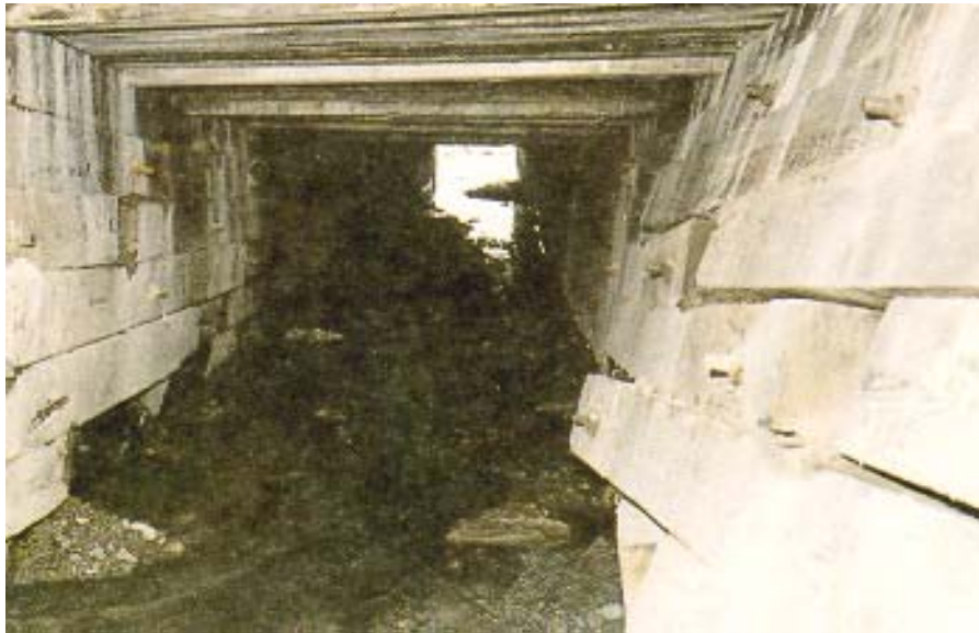
Figure 8.7(c) Wood Culvert
