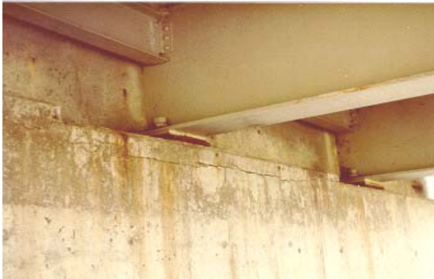
Figure 8.1(e) Concrete Abutment Wall
