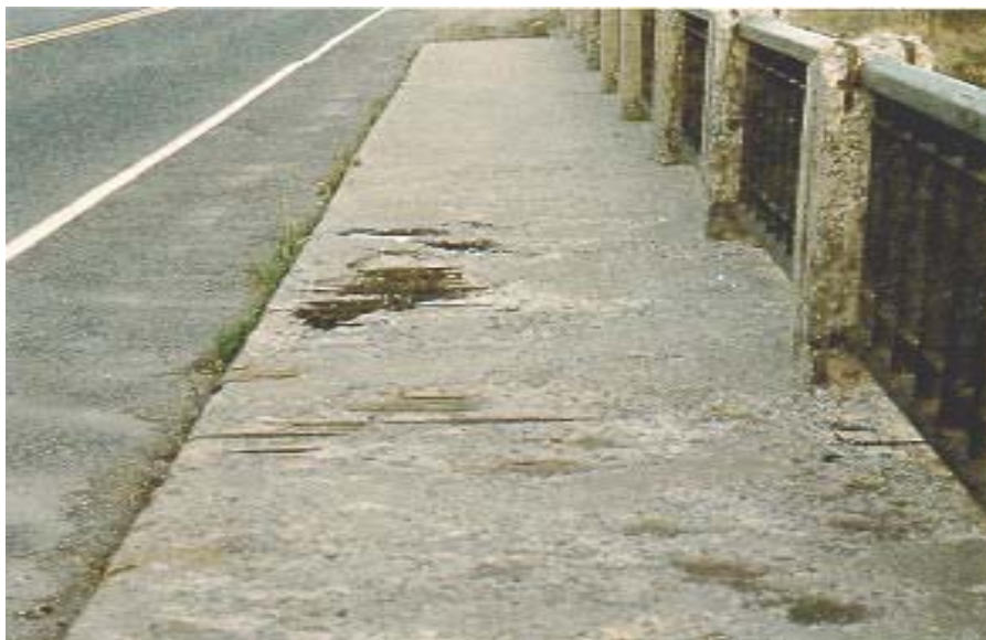
Figure 8.2(d) Concrete Sidewalk
