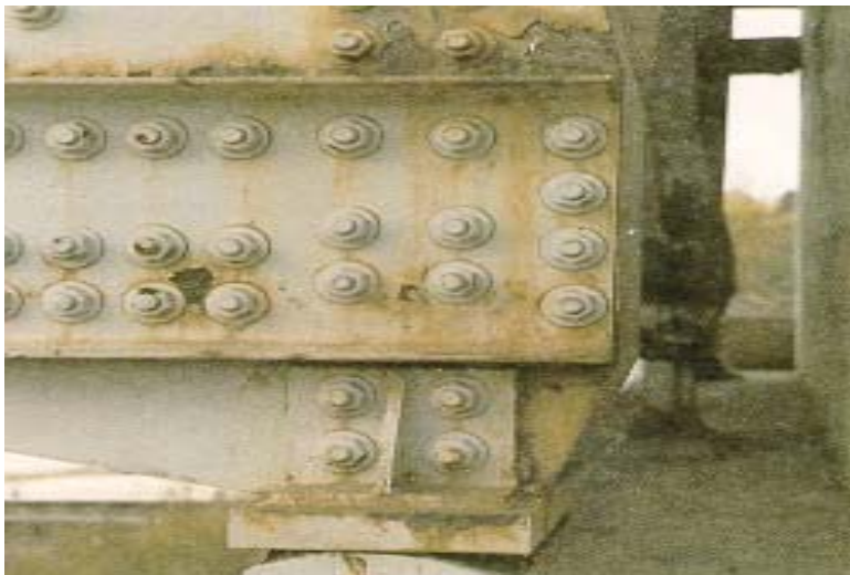
Figure 8.6(f) Truss Primary Connection at Abutment Bearing
