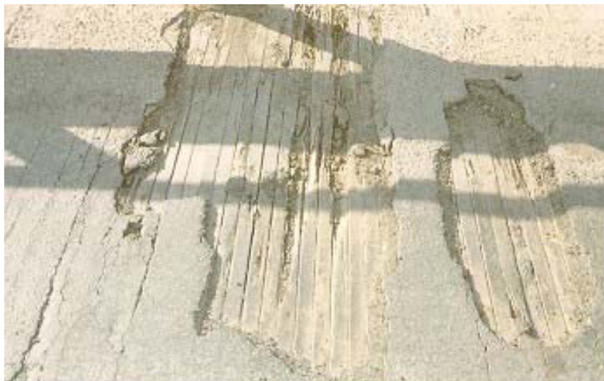
Figure 8.8(n) Asphalt Wearing Surface on Laminated Wood Deck
