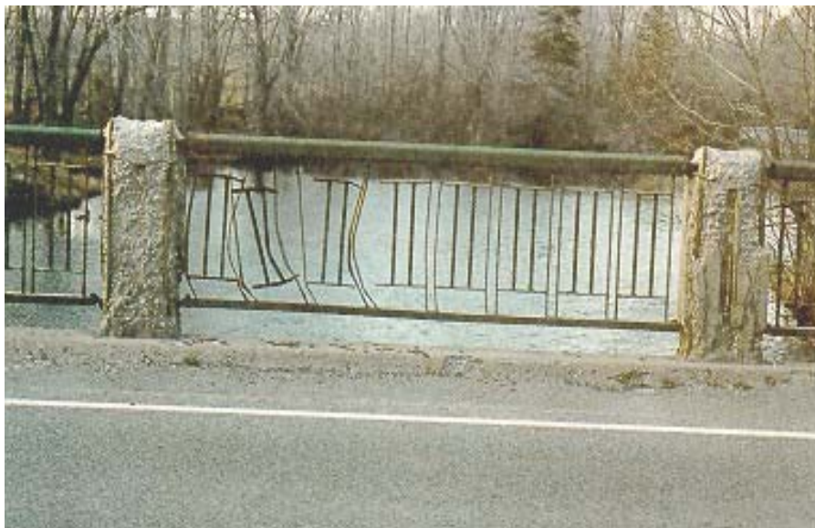
Figure 8.3(f) Steel Railing with Concrete Posts
