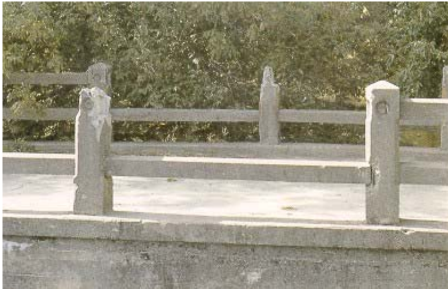
Figure 8.3(c) Concrete Railing
