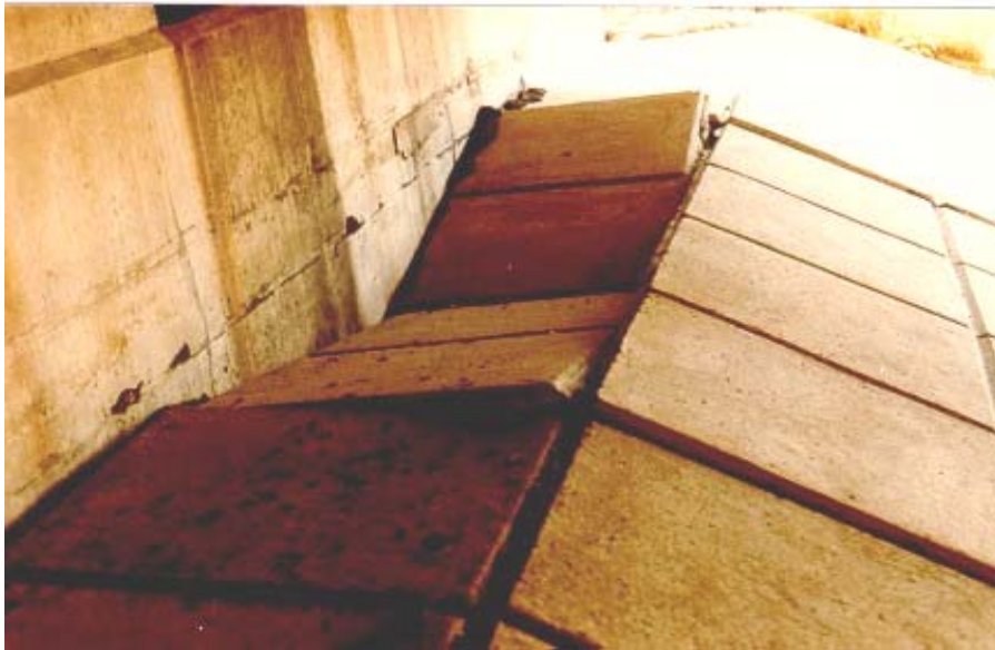
Figure 8.9(f) Cast-In-Place Concrete Slope Protection
