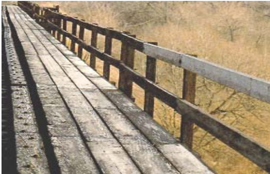
Figure 8.2(e) Wood Sidewalk
