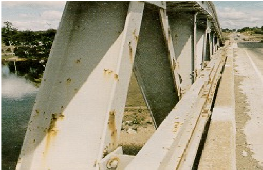
Figure 8.6(e) Steel Pony Truss
