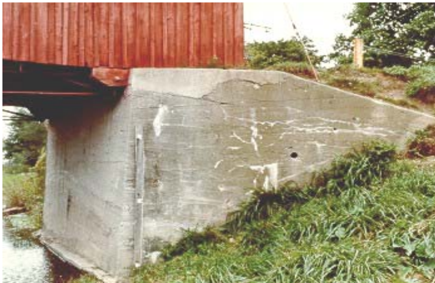
Figure 8.1(p) Concrete Wingwall
