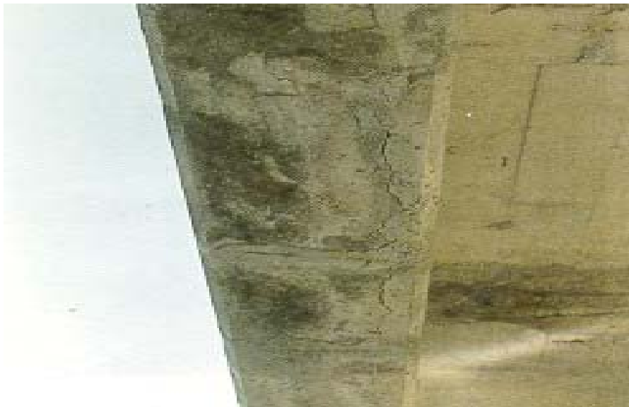
Figure 8.4(b) Reinforced Concrete Girders
