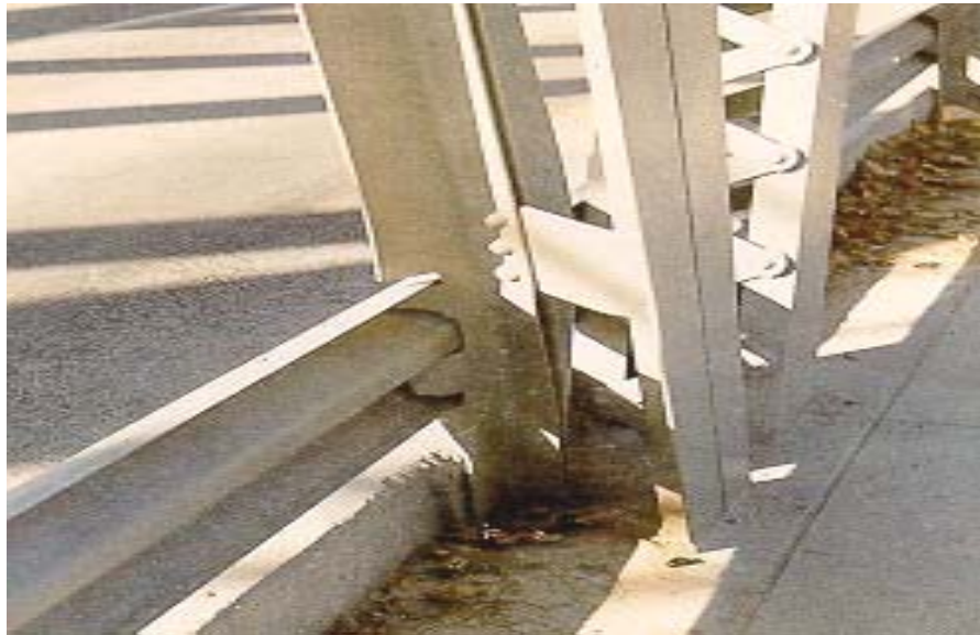
Figure 8.14(c) Vertical Member of Steel Through Truss
