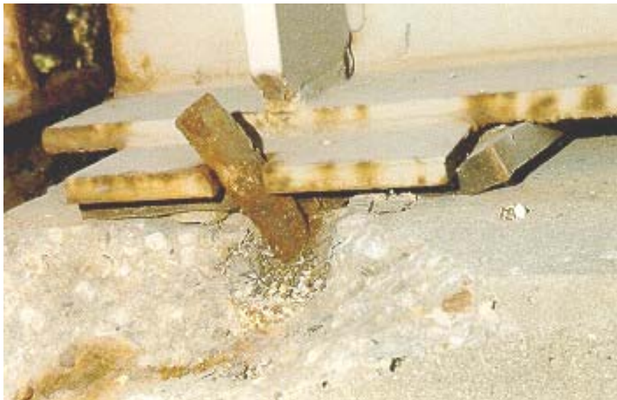
Figure 8.1(j) TFE Elastomeric Bearing
