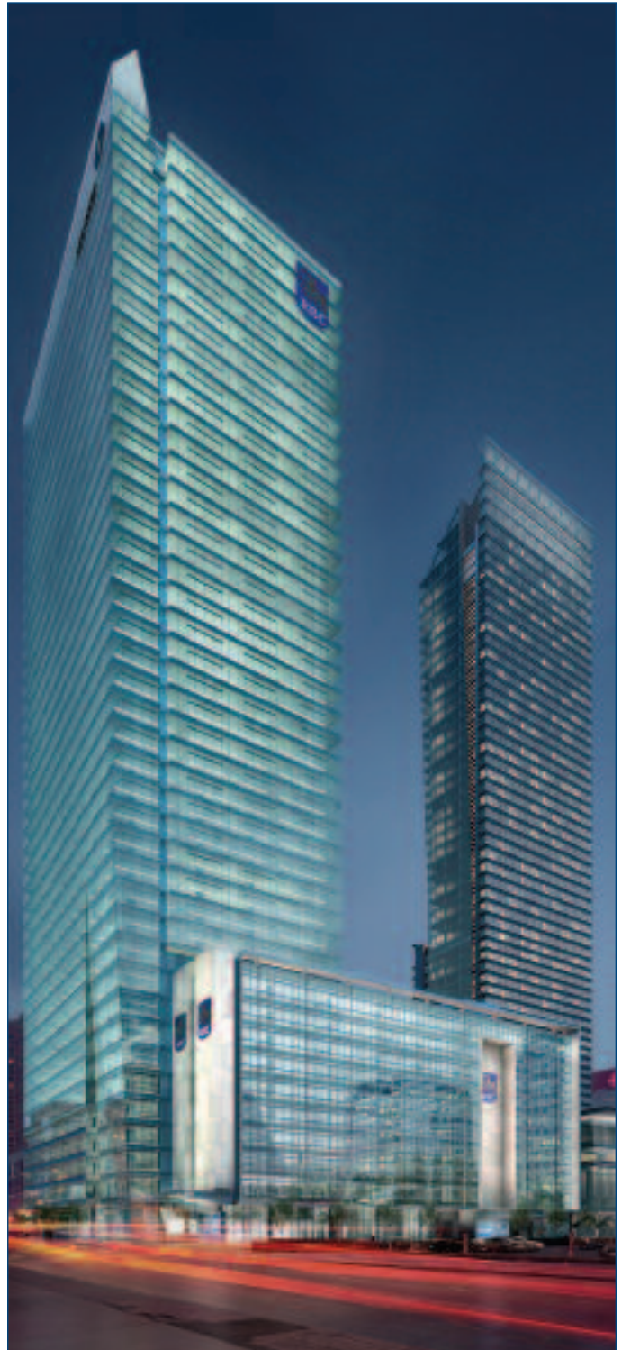
Cadillac Fairview's RBC Centre, scheduled to open in 2009, is expected to use 50 per cent less energy than buildings built to the Canadian National Energy Code.
