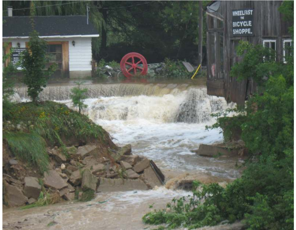
An unusual flash flood event occurred in the small community of Scone in August. The sudden onset of water over a 3 hour period overtopped the dam and flowed around the mill structure, resulting in extensive damage.
