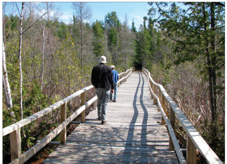
A boardwalk is rebuilt, thanks to a generous donation. It crosses over a wetland area and connects the Cedar Forest and the Camp Loop trails.
