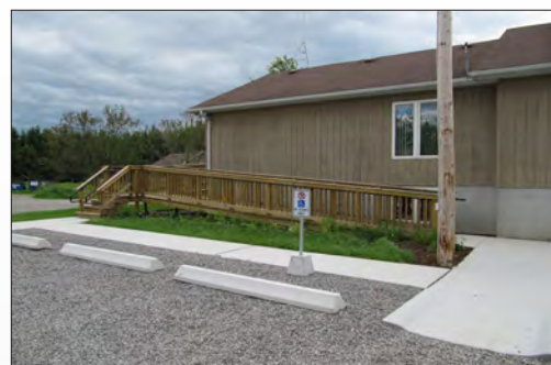
A new accessibility ramp is constructed through a grant from Human Resources and Skills Development Canada.
