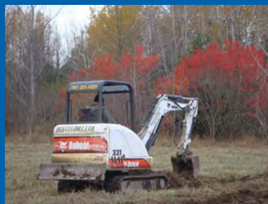
Above: Hoek Van Holland Landscaping helps smooth out the ground.
