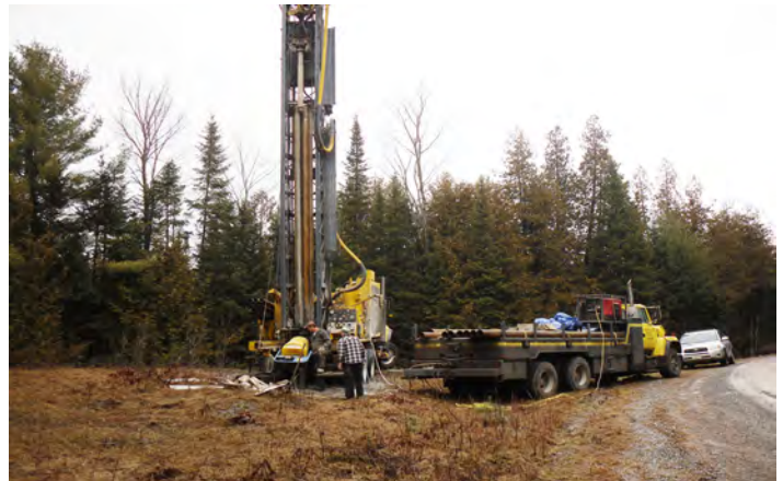
Two groundwater monitoring wells are drilled in Galway-Cavendish and Harvey.
