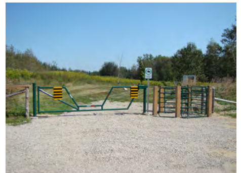
A new gate is installed at the north entrance of Durham East Cross Forest Conservation Area. It allows horses to access the trails, while preventing motorized vehicles from entering.
