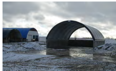
A manure storage project in the Kawartha-Haliburton Source Protection Area. By covering and situating manure on a concrete pad, nutrient runoff is significantly reduced.
