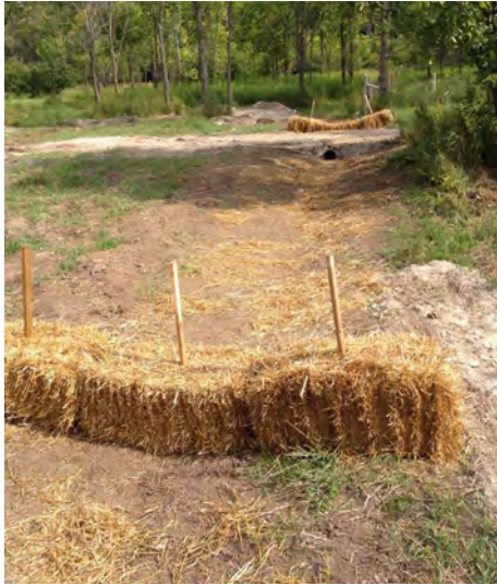
Drainage is installed at Howlers Corners to keep the site dry all year round. The off-leash park will open in June 2013
