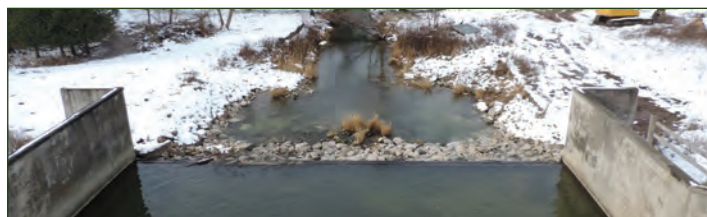
The Morrison Dam riprap reconstruction project – after completion – is shown above.
