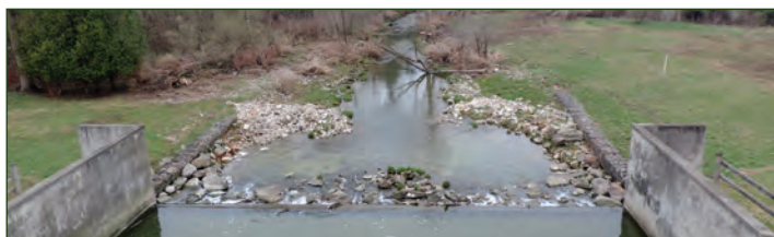
The photo above shows Morrison Dam riprap reconstruction project – before completion.
