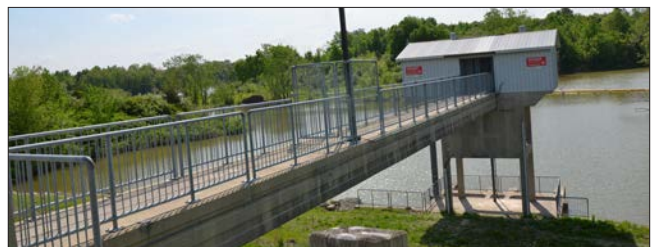
Parkhill Dam control structure.
