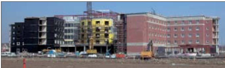
Construction to add 250 new long-term care beds at the Yee Hong Centre for Geriatric Care in Scarborough, is scheduled to finish by April 2004. The facility will serve Alzheimers and Dialysis patients within Toronto's Japanese and Chinese communities.
