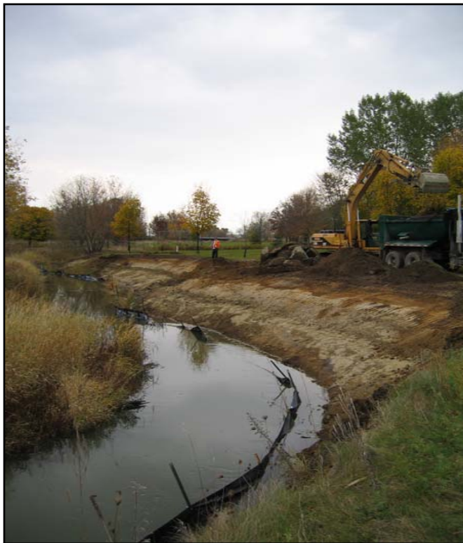
Restoring floodplain in Northwood Park, Beeton
