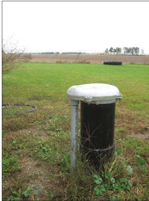
Upgraded well project
