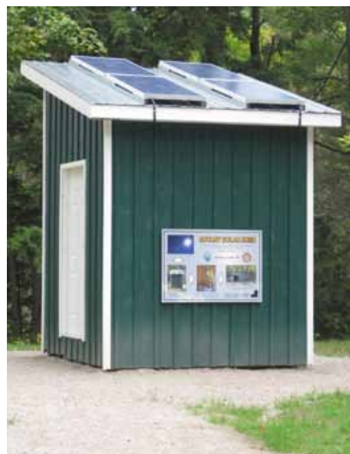
The Rotary solar shed is both functional - for powering the sugar house - and acts as a living model for educational purposes.
