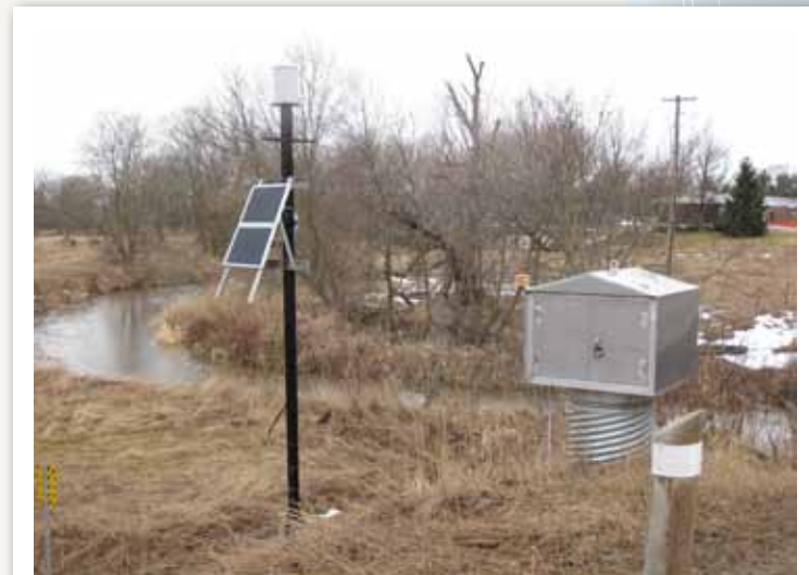
A gauge shelter on Bailey Creek near Beeton.
