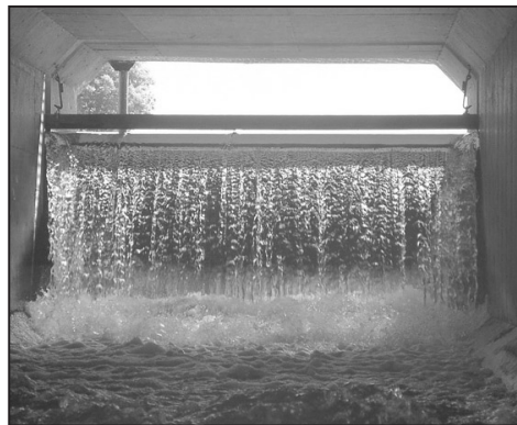
Regular maintenance of dams, such as Sydenham Dam (above) are necessary to maintain the safety and integrity of the structures. The CRCA is in the middle of a major water control structure maintenance program.
