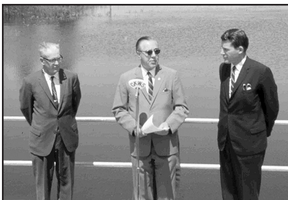
The CRCA's first project was the Broome-Runciman Dam in Brockville. Harvey Benton, Elizabethtown, Mayor John Broome, Brockville, and the Hon. James Auld, Minister of Tourism and Information officially opened the dam in June 1967.
