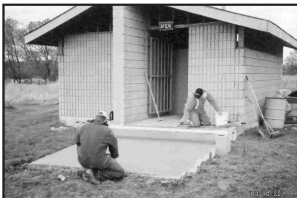
CRCA staff completed accessibility improvements to the washroom facilities at Lemoine Point Conservation Area in the fall of 2003.
