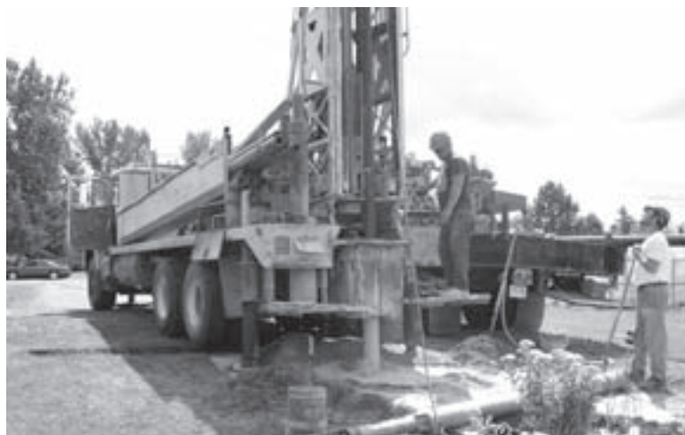
The CRCA recommends that the Clean Water Act include protection for wells, not just municipal drinking water supplies. This photo shows a new well being drilled.
