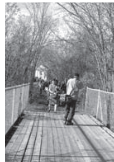
Assessing the condition of the Yarker bridge on the Cataraqui Trail is one of several projects being undertaken by Queen's University students this year.
