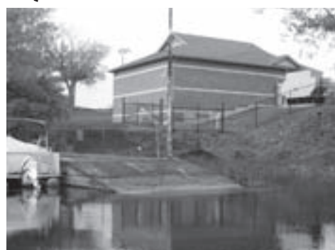
The Sydenham Water Treatment Plant is the newest plant in the Cataraqui Source Protection Area. It has been operating since July 2006.
