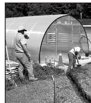
(Top) Steve Mommertz of Loyalist Irrigation poses with the Friends' Jane Murphy. (Above) Installation of an irrigation system called for all hands on deck.
