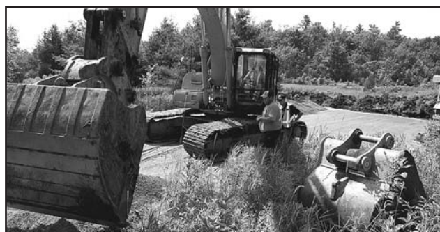
A high hoe digs a drainage ditch at the Marble Rock property near Gananoque. The new parking lot is under construction in the background.
