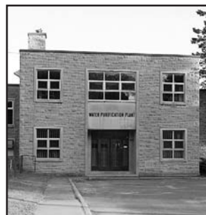
Grants to reduce potential drinking water threats are available to landowners and businesses located near municipal drinking water facilities such as the Kingston Central Water Intake shown here.
