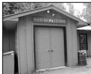
The Nature Centre at Mac Johnson Wildlife Area is used for school programs, meetings and community events. A new facility is being considered by the CRCA.
