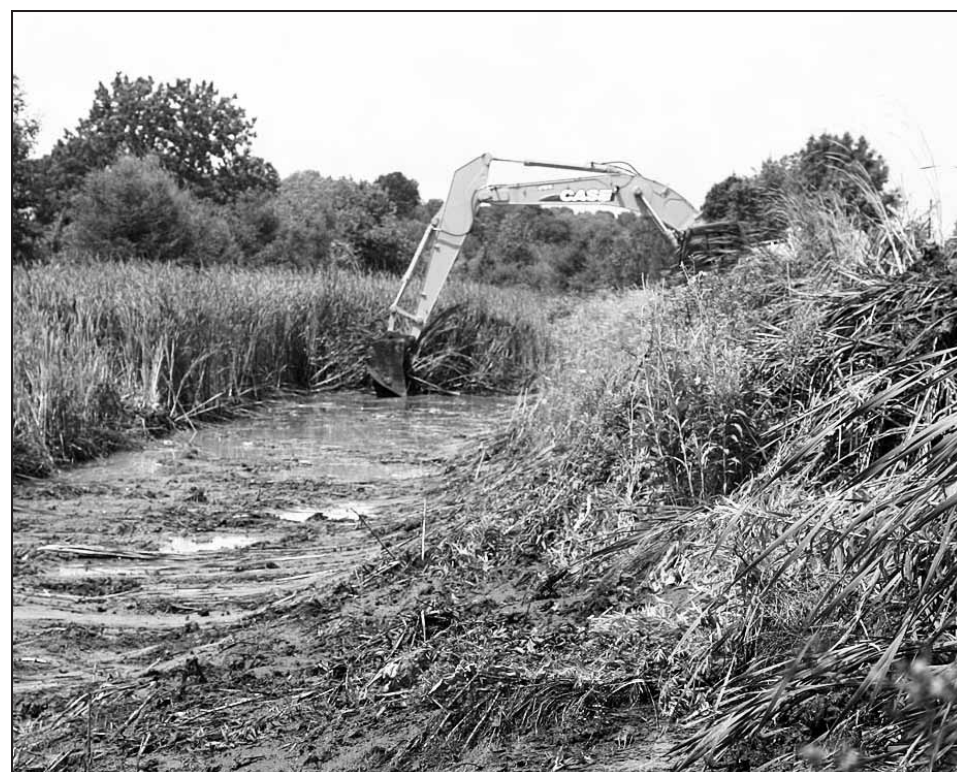
Regular maintenance of the Brockville Detention Basin is required to make sure that it can continue to perform its flood control function. Here sediment and vegetation are being removed to restore the capacity of the detention basin.
