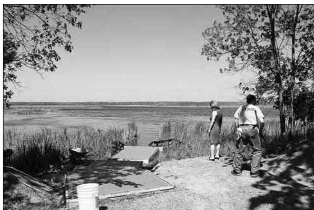
Taken at the beginning of June, this photo shows the newly-poured concrete steps at the Mac Johnson Wildlife Area canoe launch.
