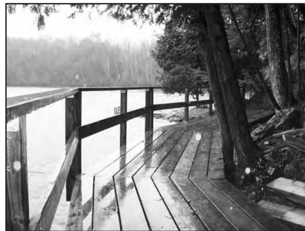
A new boardwalk along the shore of Gould Lake will provide safe access from the beach area to the swimming dock. The boardwalk was built by CRCA staff with a lot of help from Rideau Trail Association volunteers.
