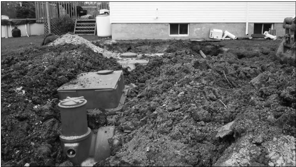
Septic system upgrades were one of the most funded projects under the Ontario Drinking Water Stewardship Program. This photo shows a new septic system being installed.
