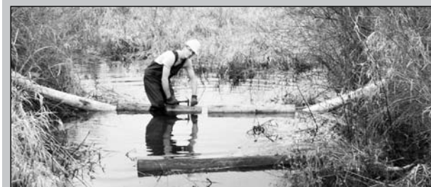
CRCA Watershed Engineering Technologist Shawn Fairbank installs a flotation boom in the Brockville Detention Basin.
