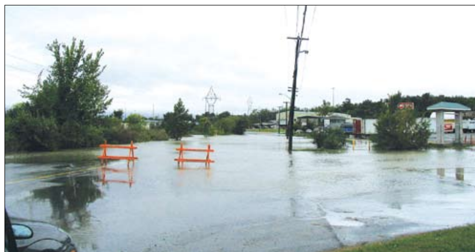
Extreme rainfall events such as the end of Hurricane Frances in 2004 in Kingston can cause streets to flood. This is because storm sewers and other infrastructure cannot handle the large flows and runoff that occur suddenly.
