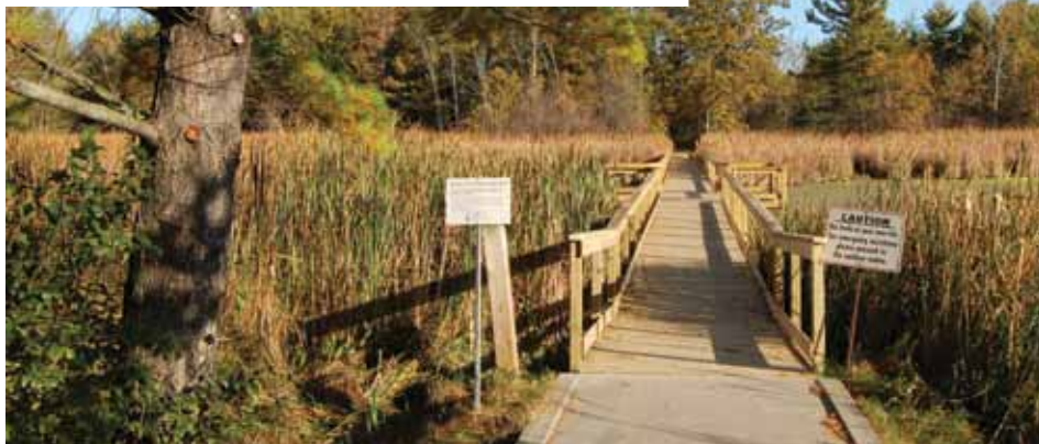
A new boardwalk was built over the summer at Little Cataraqui Creek Conservation Area. It was complete and ready to use by the fall.
