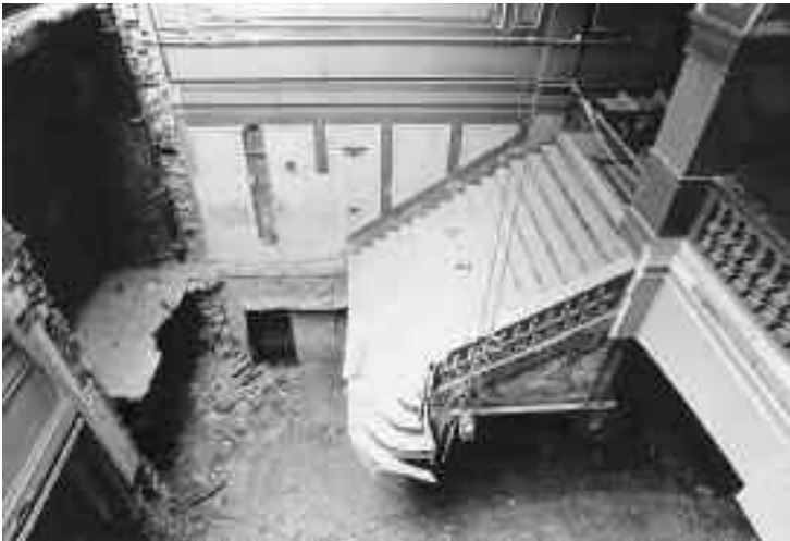
The Elgin and Winter Garden Theatre Centre (Toronto). In 1987, a basement is excavated under the lobby corridor, and the grand staircase is suspended in the air.
