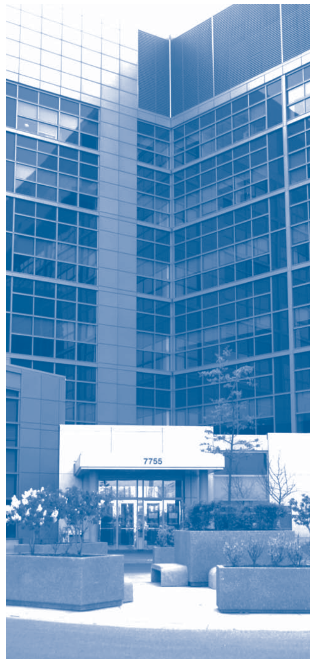
A. Grenville & William Davis Courthouse, Brampton
