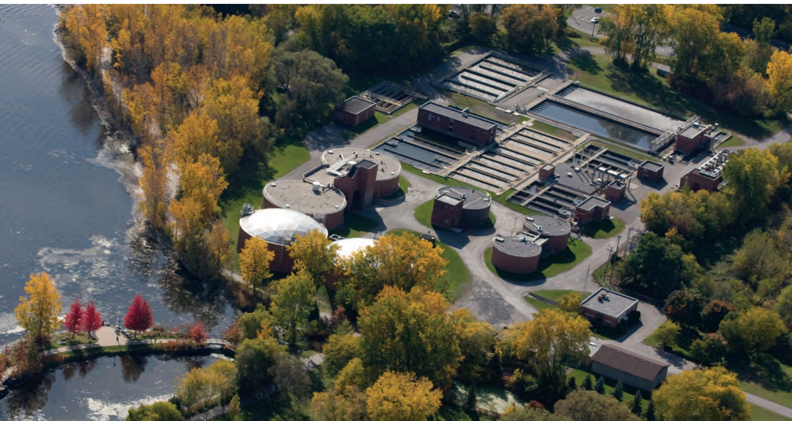
Belleville Wastewater Treatment Plant
