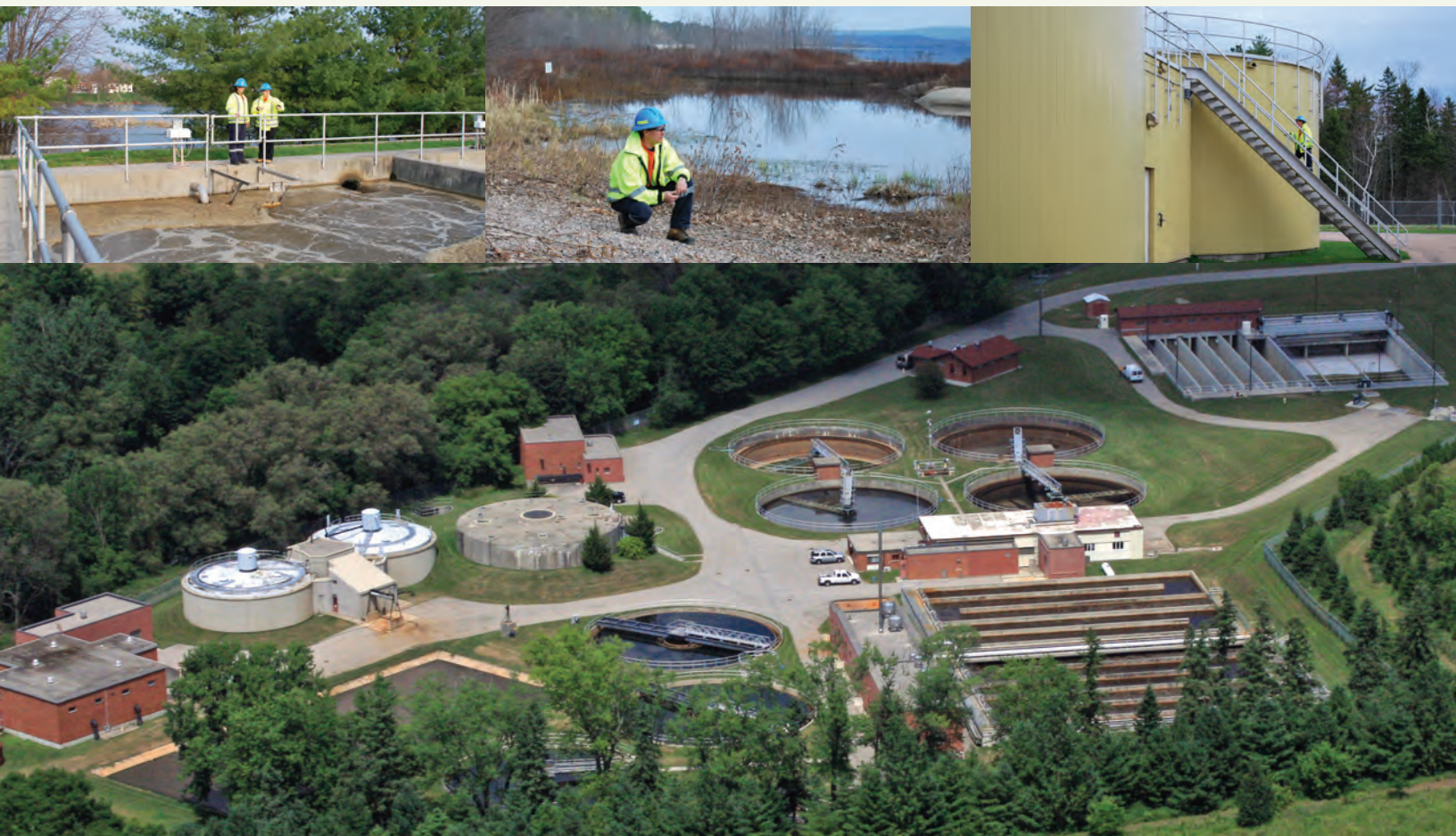
Stratford Wastewater Treatment Plant
