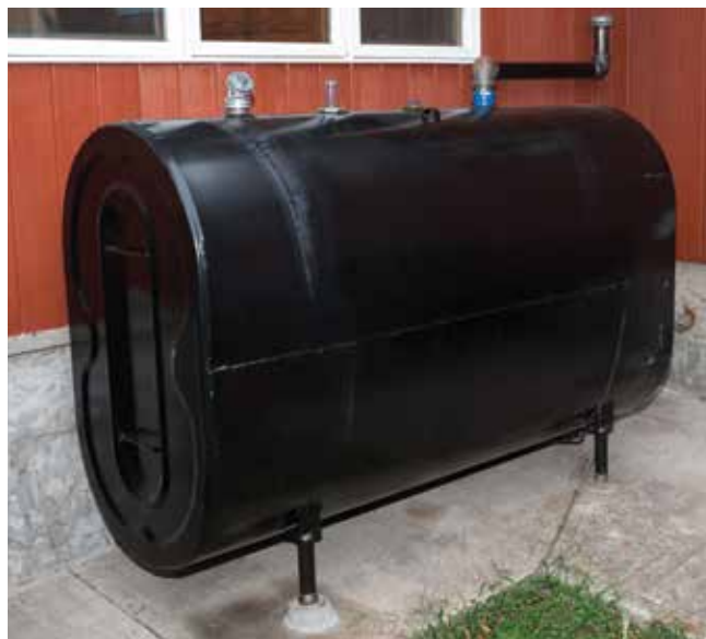
Example of outdoor above-grade fuel storage tank.
