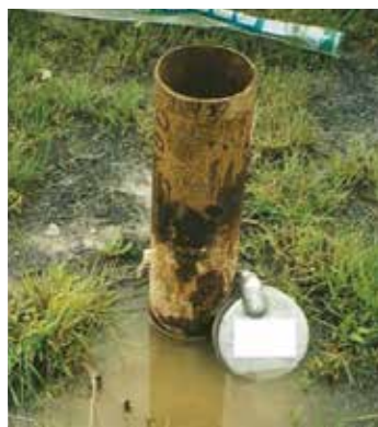
Poorly maintained water supply well.
