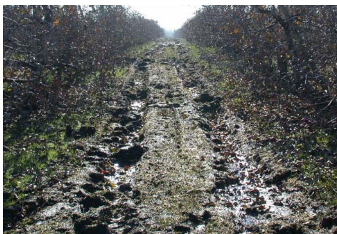
Figure 1. Side hill seep contributed to this rutting in 2006. Consider grading and further drainage to reduce the problem for the future.
