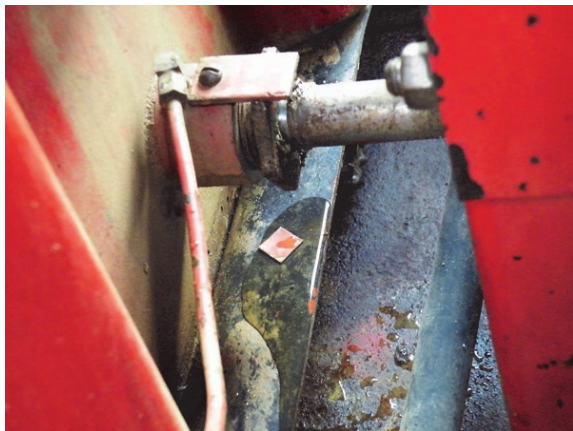
Figure 12: A leaky mechanical agitator – a little is alright, but a lot means you have to tighten or even repack the gland.
