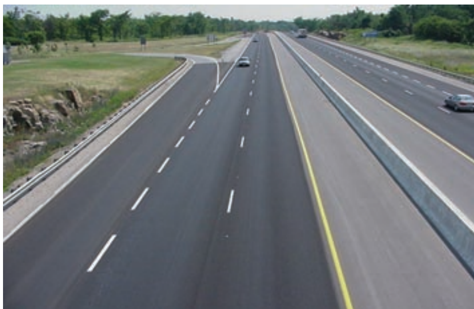
Microsurfacing Application: Highway 401 at Ganonoque.
