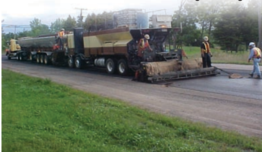
Microsurfacing Train: Showing Nurse Truck and Microsurfacing Truck
