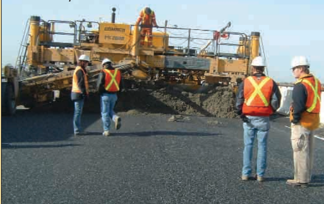
Shawn McGuire and Ken Brisbois in the foreground observe project that widens over 13 km of Hwy. 401 between Hwy. 77 and Essex Road #42
