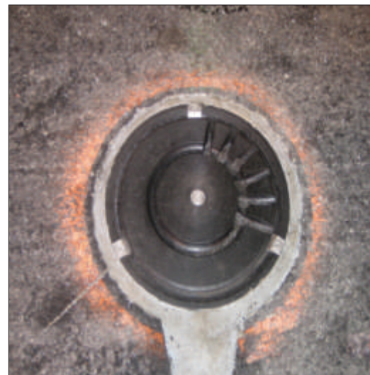
Above: FAST nozzle embedded in the pavement of the ramp and tunnel.
