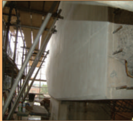
ABOVE: SCC surface finish of the Garden City Skyway pier.
