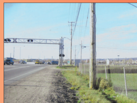
North Bay Highway 11/17 Bypass looking north at ONR crossing. Congestion has been a major issue associated with the crossing.
