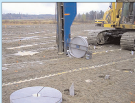
Figure 2. Spools of wick drain pushed into the ground
