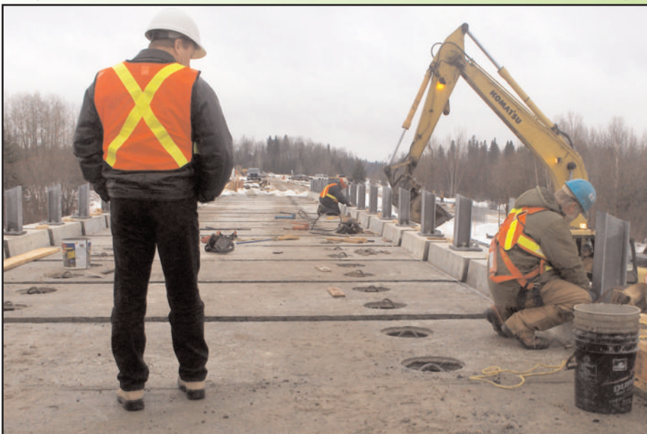
Figure 1. Full depth and full roadway width deck panels used for the new Passe-à-Fontaine Bridge
