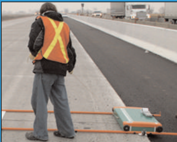
Figure 1. MTO Staff scan dowel bar position, Highway 401
