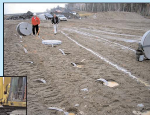
Figure 1. Grid patterned wick installation
