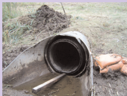
Fig.2. Highway 403 culvert with plastic liner, prior to grouting operation.
