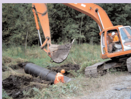
Fig 1. HDPE liner inserted through temporary backslope on Highway 403.
