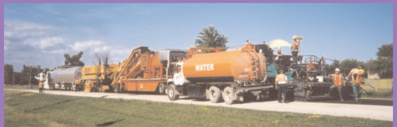
Cold in-place recycled expanded asphalt train, consisting of hot asphalt tanker, milling unit, mixing unit, and paver.
