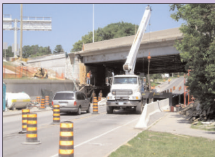
The old Island Park Bridge.
