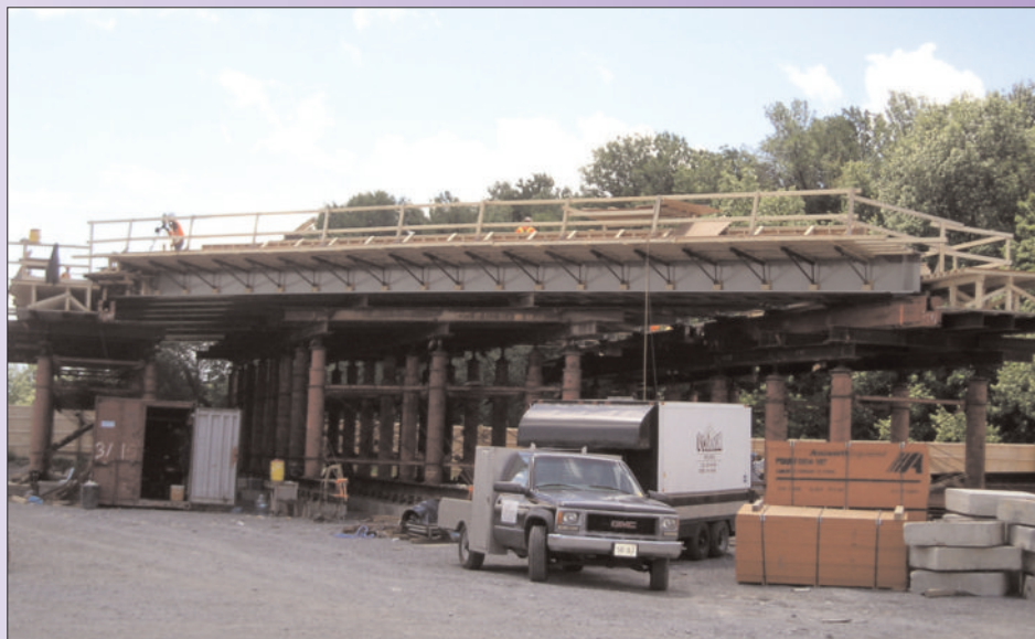
The new Island Park bridge deck under construction in the staging area.
