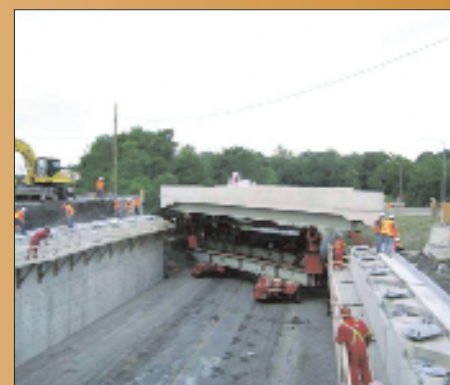
Figure 2: A Self Propelled Modular Transporter (SPMT) carries a bridge deck from the staging area to the final site.
