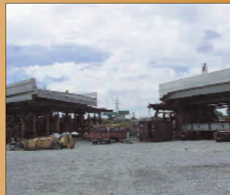
Figure 1: The new Island Park Bridge under construction in the staging area.
