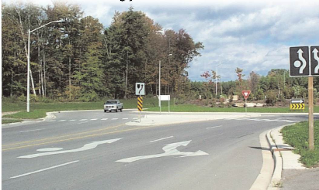
Entrance of a newly constructed roundabout
