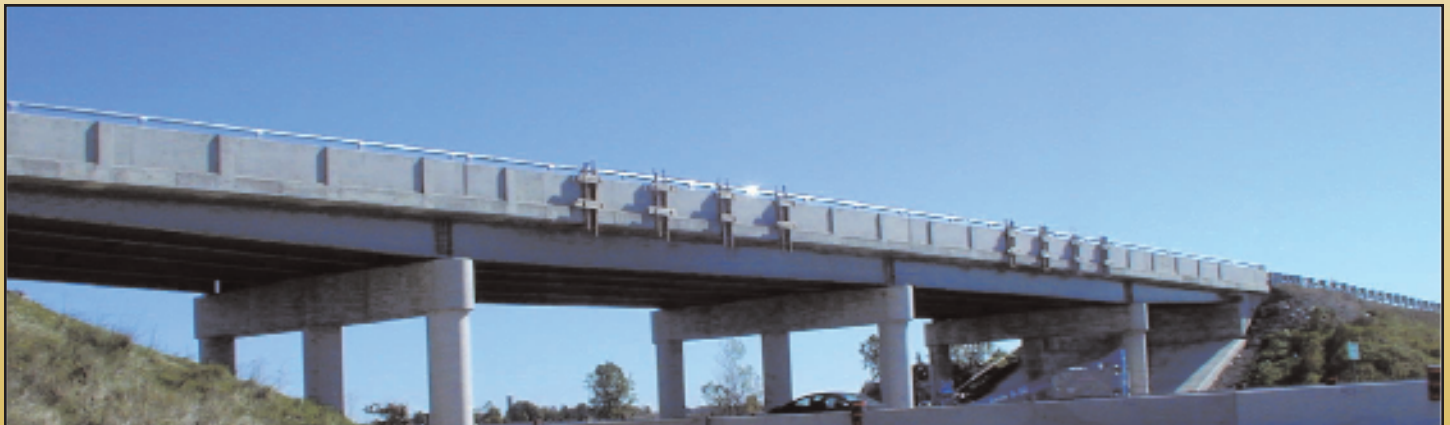
Figure 2: The completed Mull Road underpass
