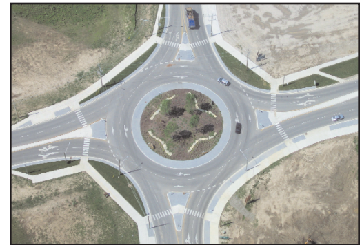
Aerial view of a roundabout with 4 intersections
