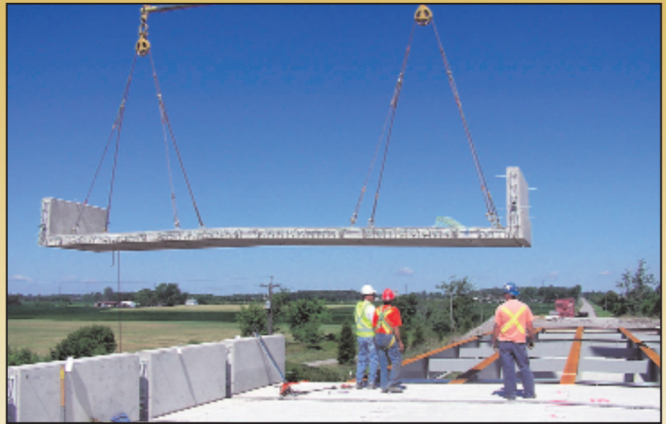
Figure 1: Workers replace the deck of the underpass using prefabricated panels
