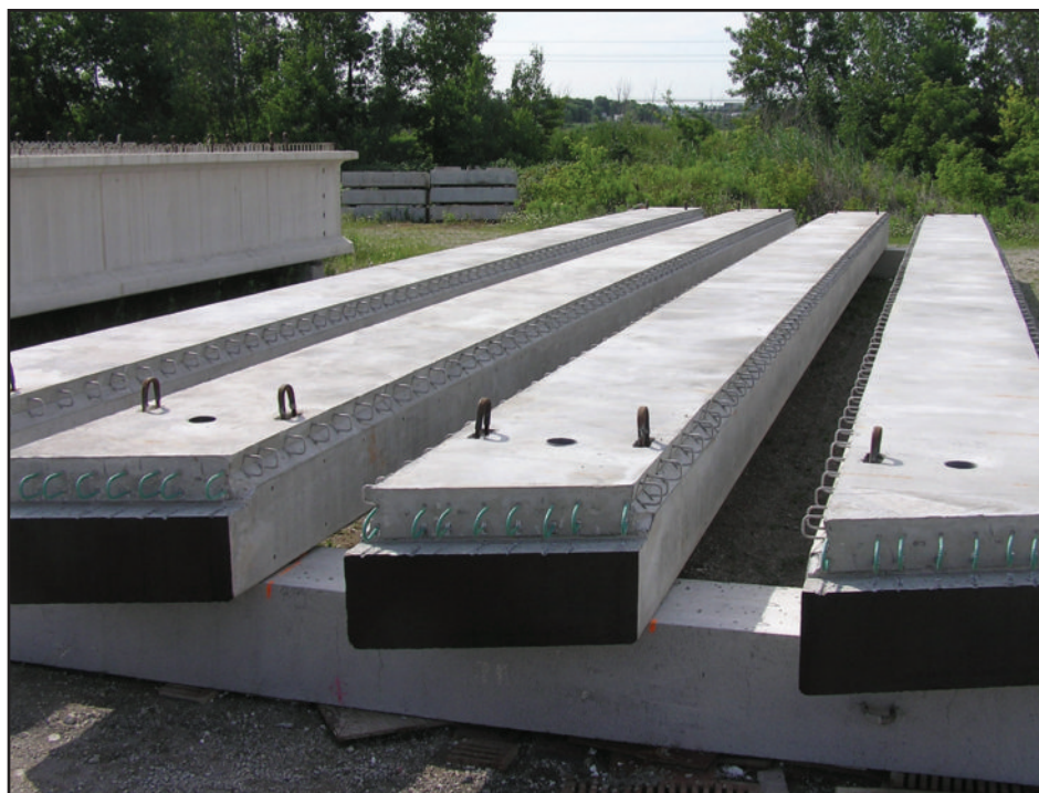
Pre-cast box girders ready for shipment to the bridge site.
