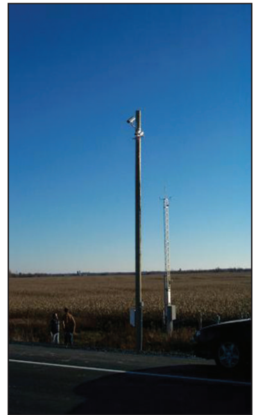
Next generation RWIS sensors detect pavement contaminants, including snow, frost, ice, and slush.
