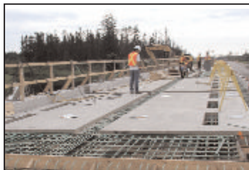
Little Savanne River Bridge, Hwy 17 Pre-cast full-depth deck panels.
