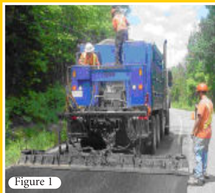
Figure 1: Placement of slurry seal by truck mounted paver.
