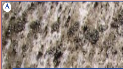
A & C: Sand particles melt down into the snow and freeze on the road, creating patterns of sandpaper-like texture on the road surface
