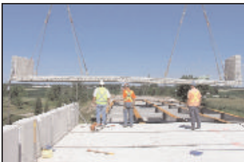
Hwy 401/ Mull Road Underpass Pre-cast full-depth full-width deck-panels.
