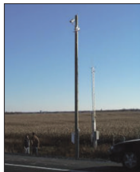
Figure 1: A next generation RWIS sensor is used to detect road weather surface conditions.
