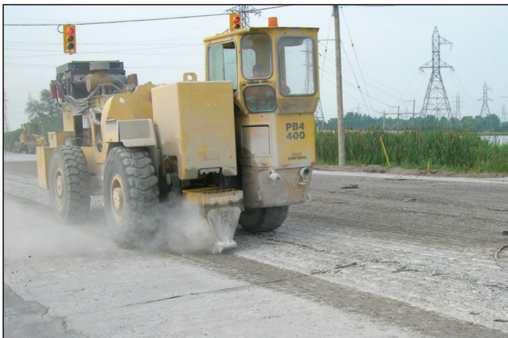
In-place resonant rubblizing uses a 44 Hz frequency on a 200 mm shoe to precisely shatter concrete pavement.
