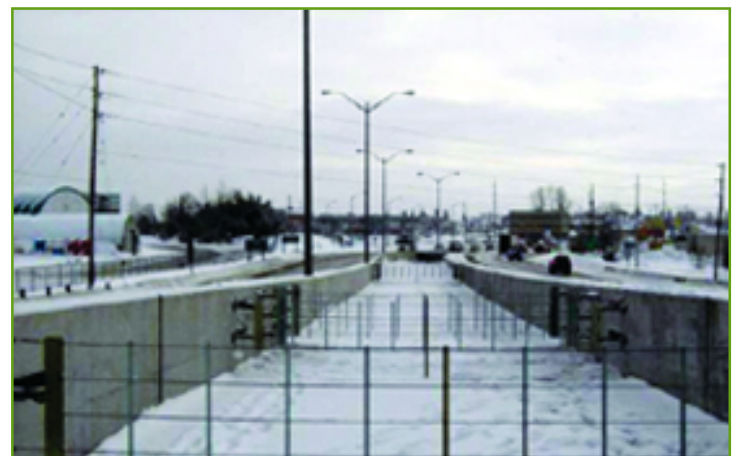
Runaway truck ramp dragnet system.
